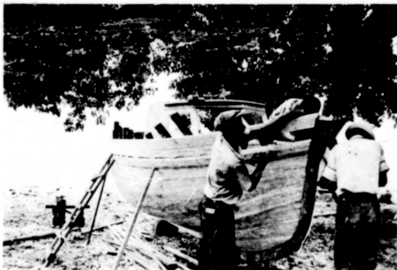
Fig. 7. Launch under construction at Half-Moon Fort (North of Speightstown), Barbados.
