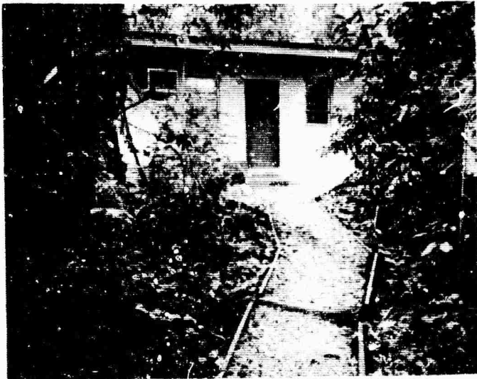
Observer and Recording System Building
