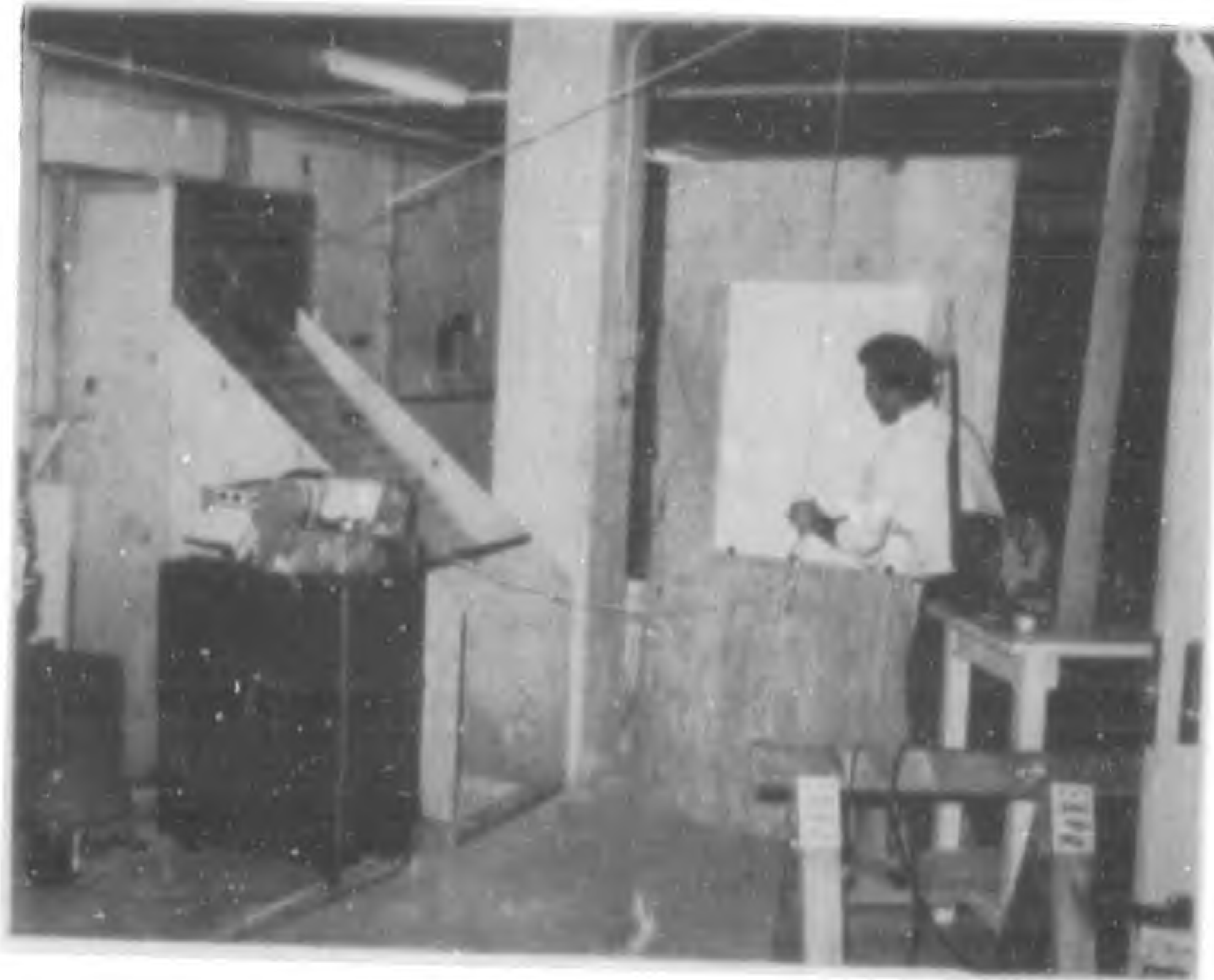
Figure 3.21 Test arrangement for horsepower measurement six foot full door punkah.
