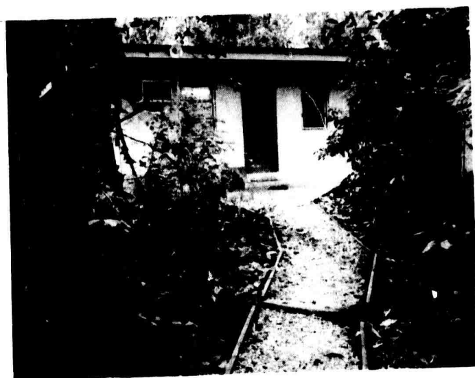
Observer and Recording System Building
