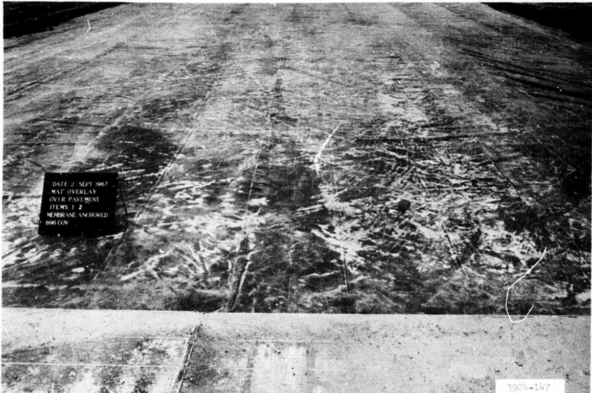
Photograph 47. T16 membrane on items 1 and 2 after secondary construction II
