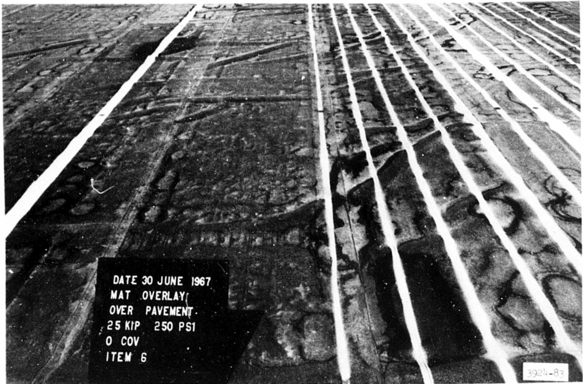
Photograph 15. Item 6 prior to traffic
