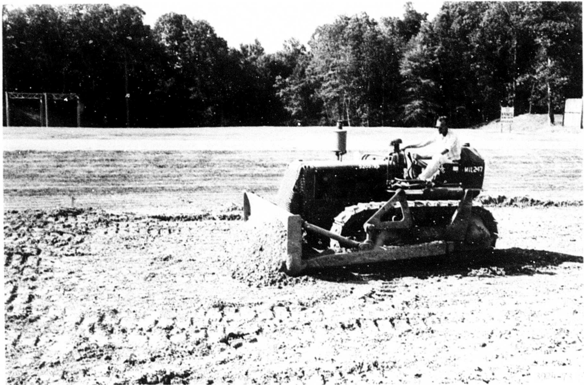
Photograph 4. Spreading clay gravel in items 3 and 4 with bulldozer
