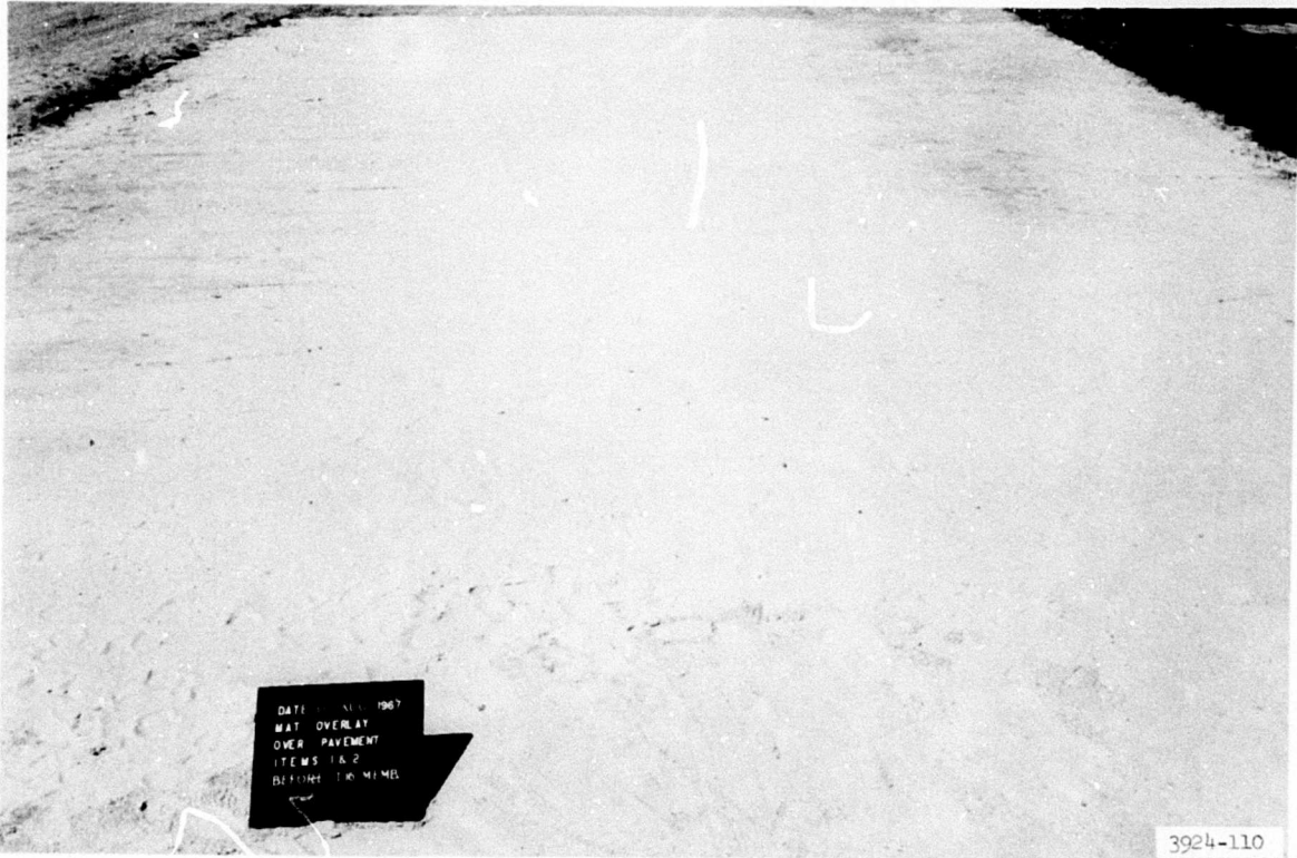
Photograph 31. Sand in items 1 and 2 after secondary construction I
