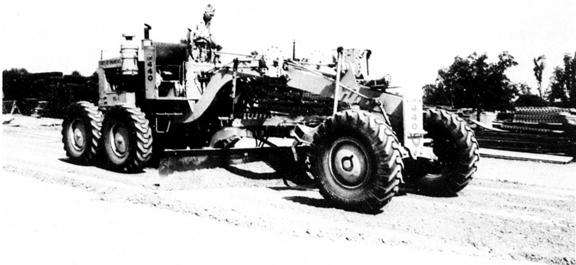
Photograph 6. Cutting lean clay to final grade with road grader
