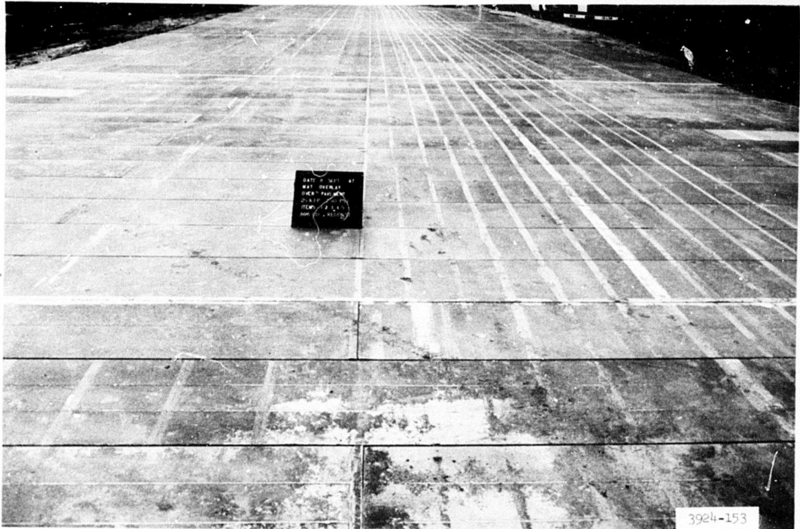
Photograph 50. General view of test section after completion of secondary construction II
