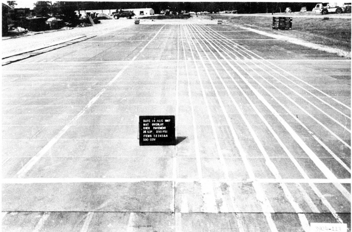
Photograph 36. General view of test section after completion of secondary construction I
