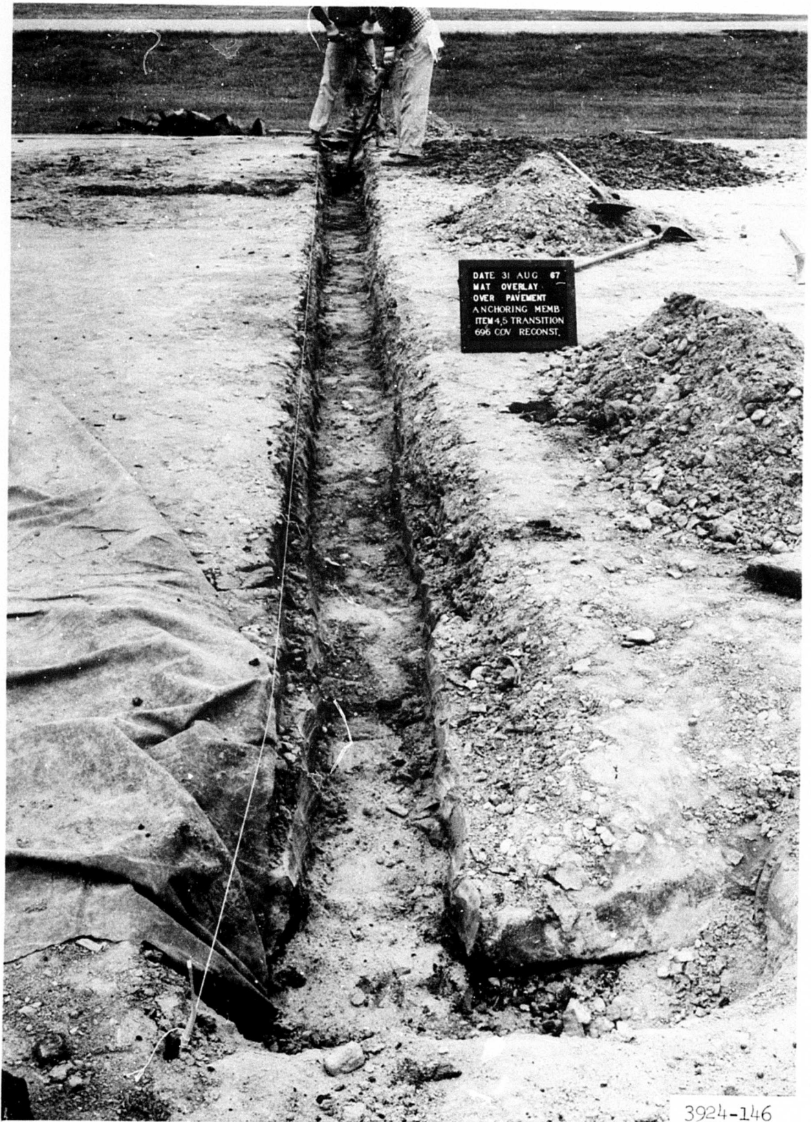
Photograph 49. Anchor trench cut laterally between items 4 and 5 in secondary construction II
