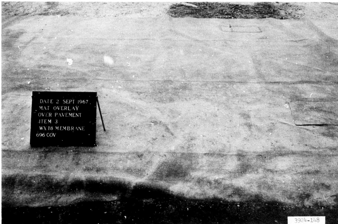
Photograph 48. WX18 membrane on item 3 after secondary construction II
