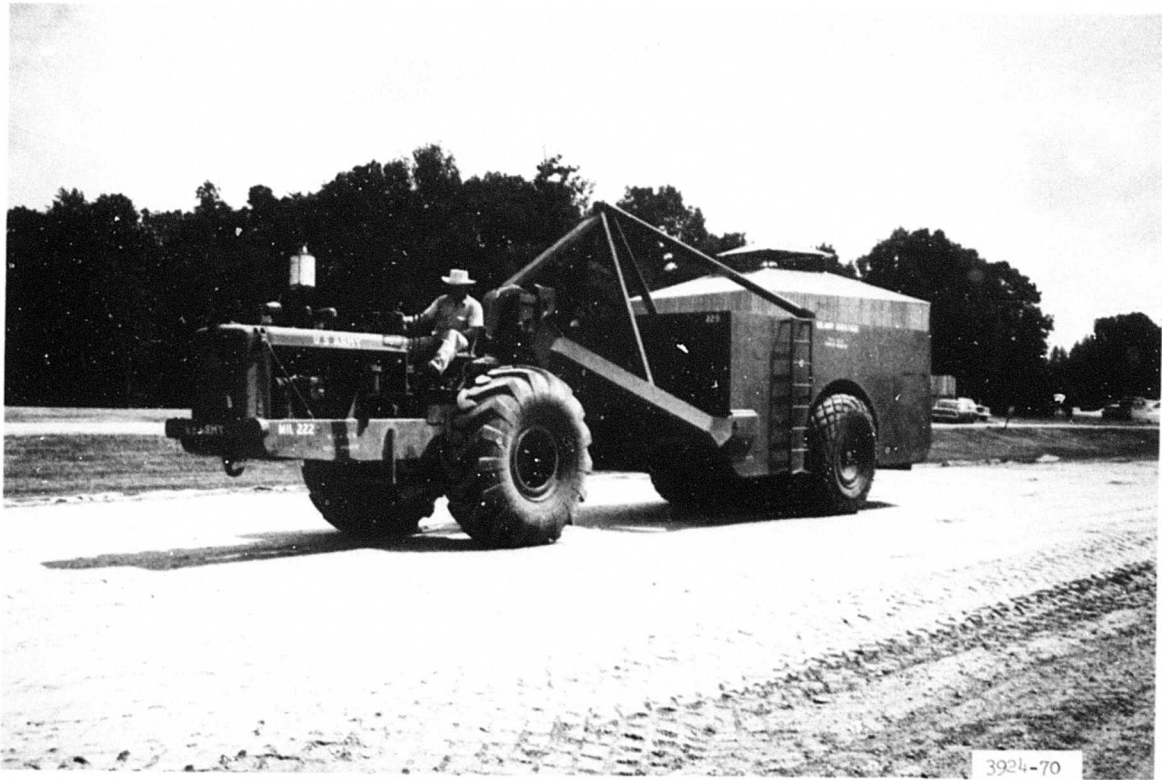
Photograph 5. Compacting clay gravel with 50,000-lb towed roller
