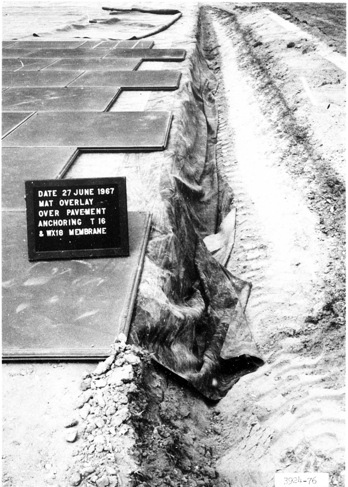
Photograph 7. Edges of membrane placed in anchor trench prior to pinning and backfilling
