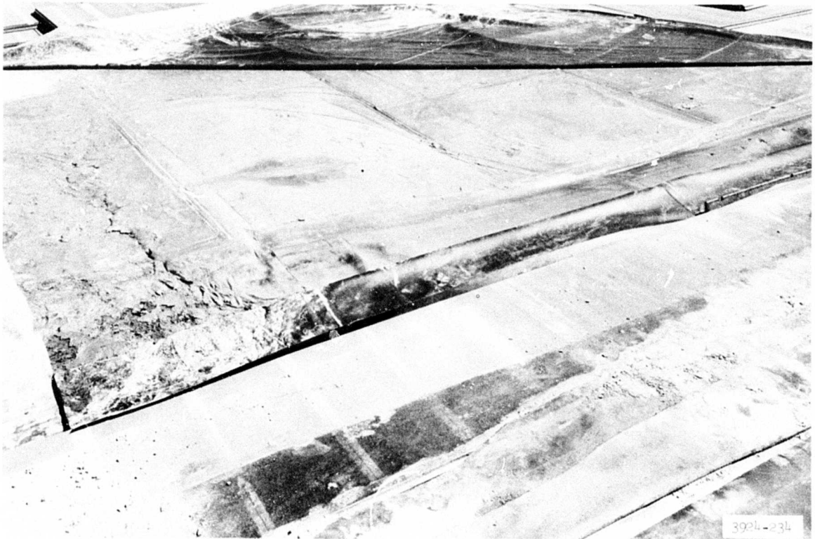
Photograph 51. Condition of soil under failed panel of XM19 (1850 coverages)
