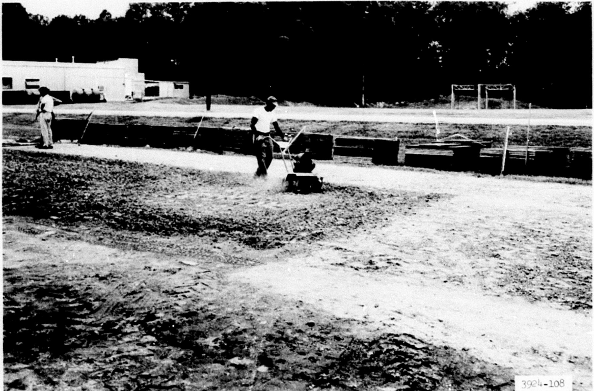
Photograph 34. Mixing cement into soil with a rotary tiller
