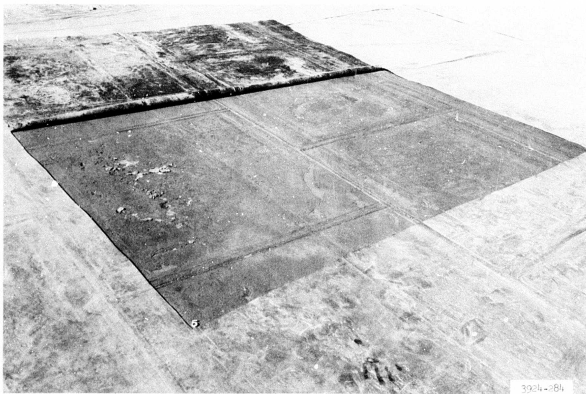
Photograph 65. Stable condition of lean clay considered typical of item 5
