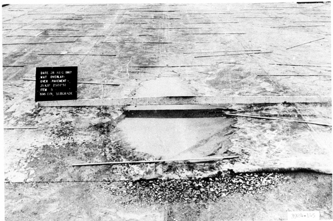
Photograph 46. Washed clay gravel between items 4 and 5 (rods are XM19 connector bars)
