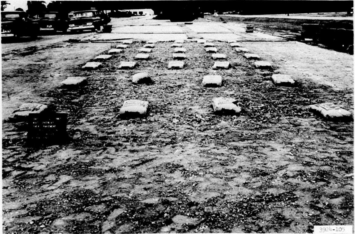
Photograph 33. Bags of cement on section preparatory to stabilizing clay gravel
