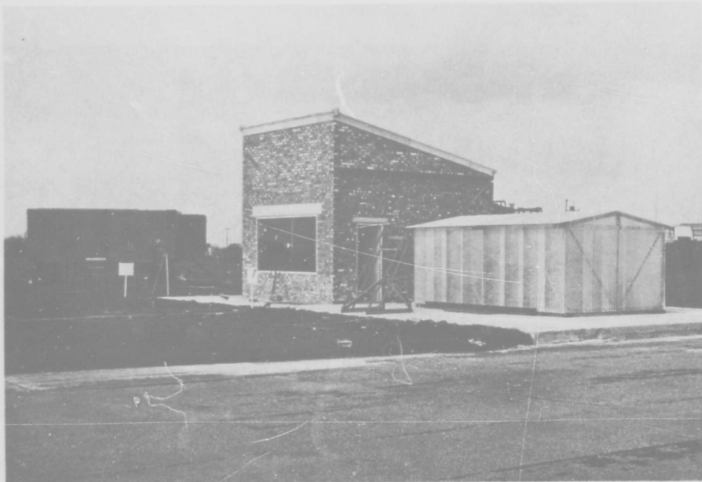
Fig.11. View of test building
