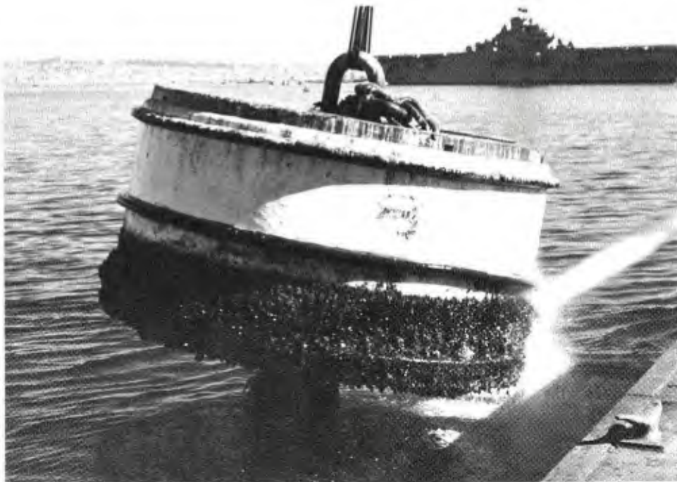
Figure 3. Hosing of marine fouling from spray-up buoy in San Diego Bay.
