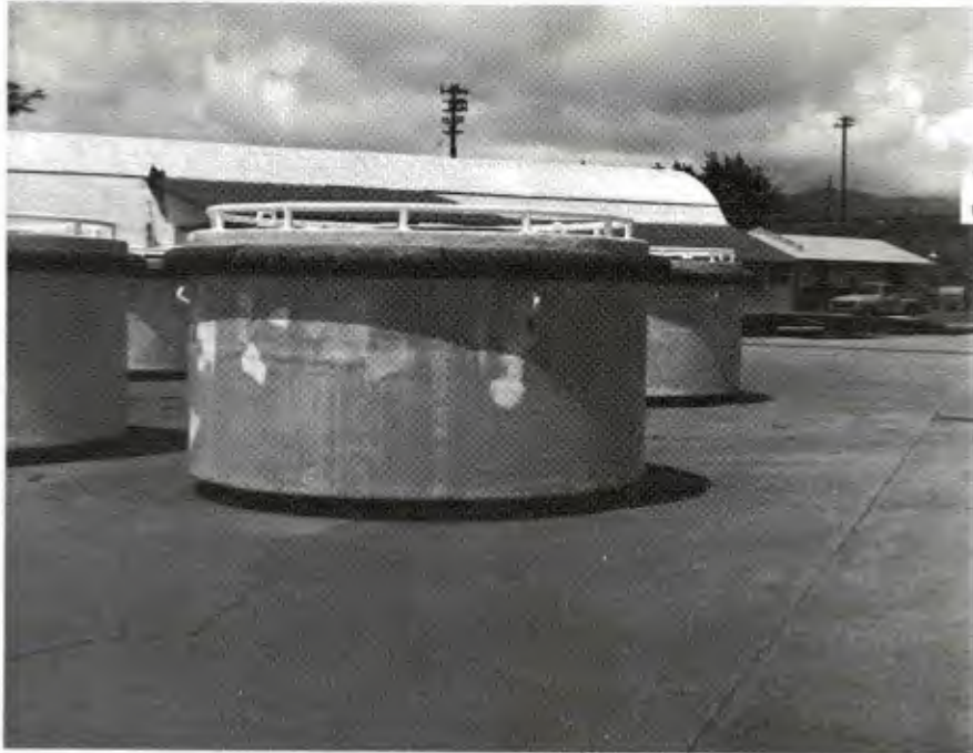
Figure 8. Steel mooring buoys at Pearl Harbor with yellowed fiberglass-reinforced polyester coating.
