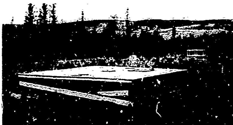
Figure III-19. Area 3 Test Building No. 6 with wood floor completed. Not to be skirted. September 1946
