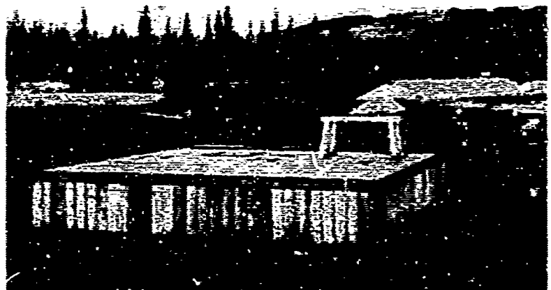
Figure III-20. Area 3 Test Building No. 7 with floor completed and skirting in place September 1946
