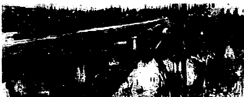
Figure I-14. Utilidor for outfall sewer line, placed on posts with crossbeams and on crossbeams on the ground surface. Noticeable settlement may be attributed to improper construction by not placing the posts to adequate depths in permafrost
