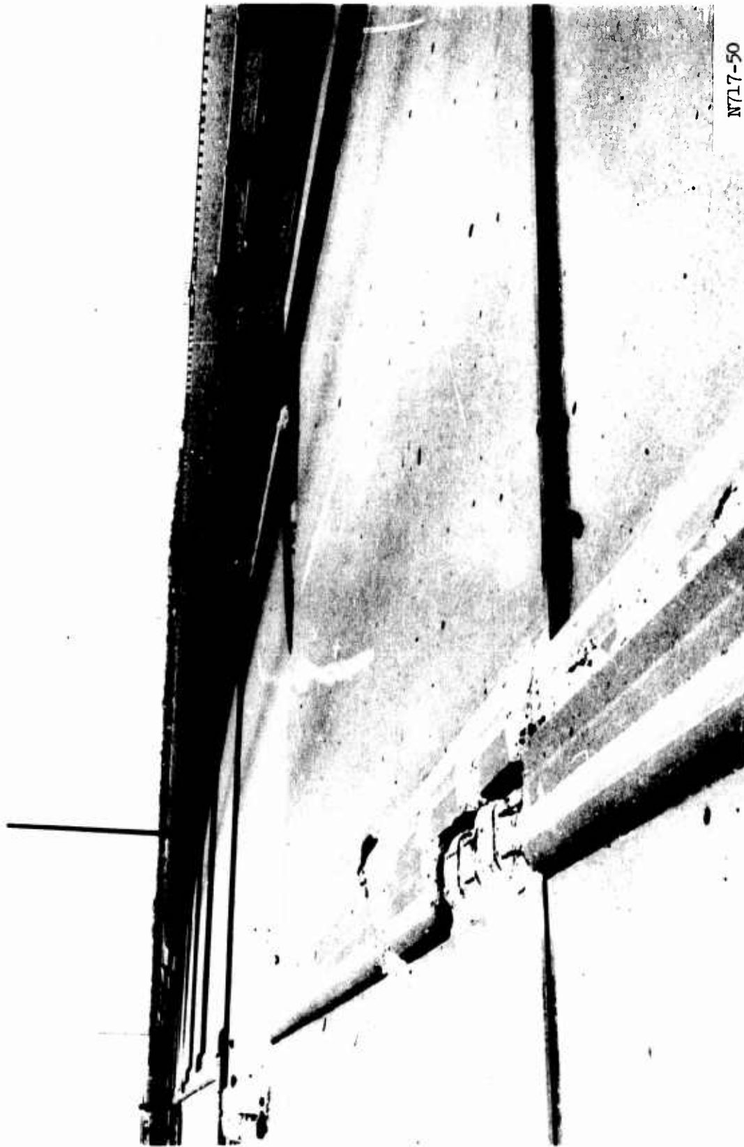
Figure 3.54 Displaced span of Bay Saint Louis Bridge.
