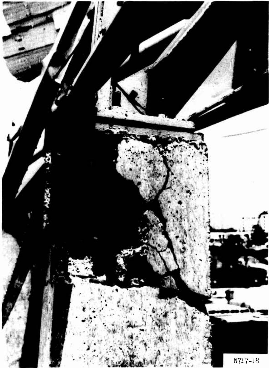
Figure 3.15 Center pier supporting west end of arch, Marine Life.
