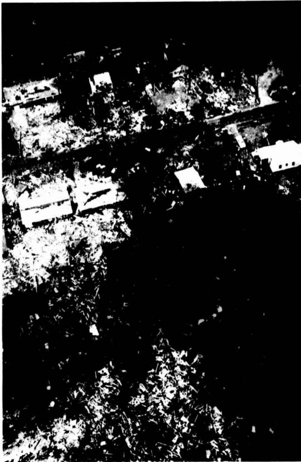
Figure 2.17 Residences and debris line in west Gulfport, Mississippi.
