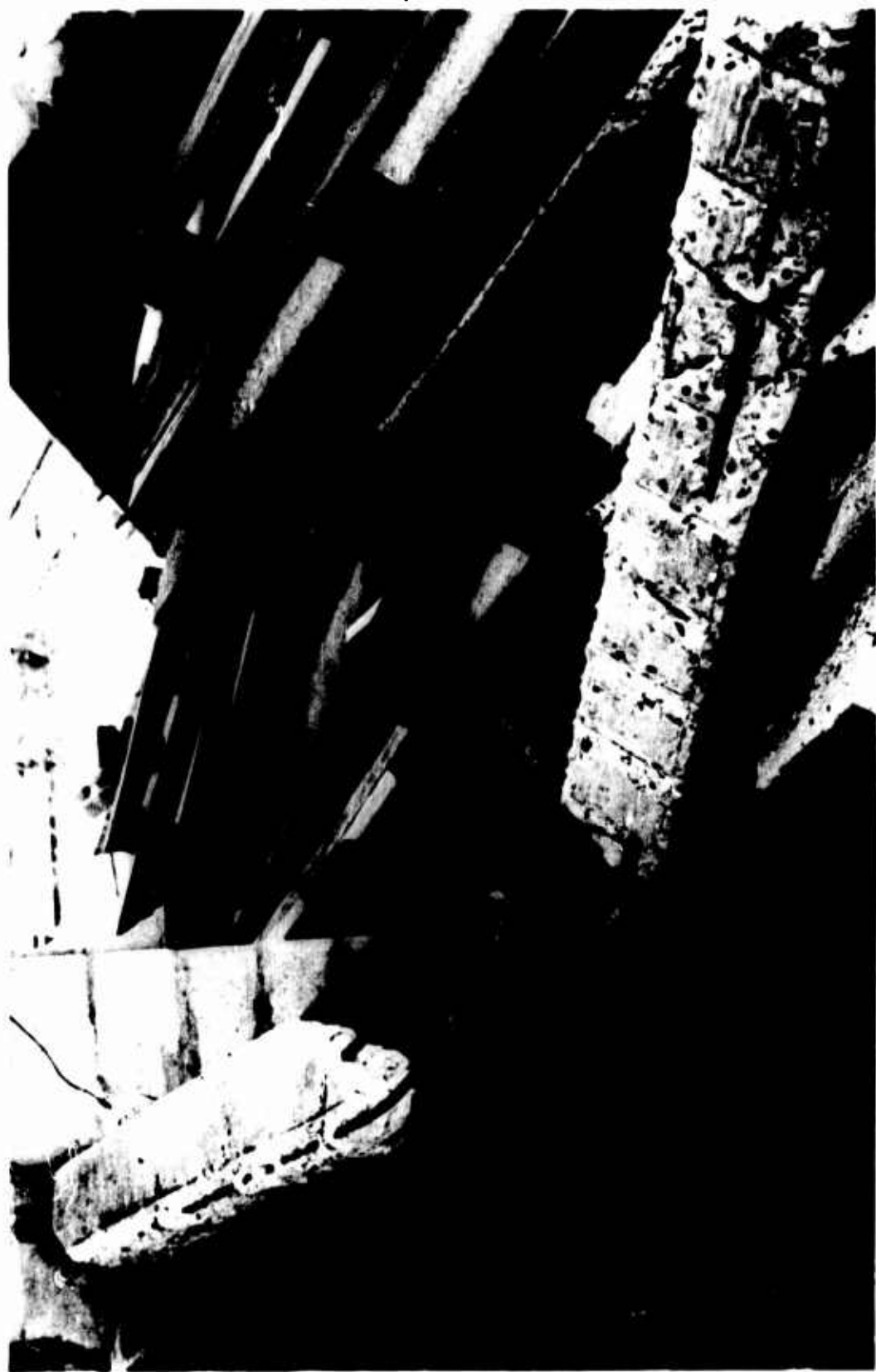
Figure 3.23 Beam failed in torsion, seating area of Marine Life.
