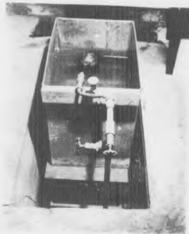
Figure 2. ball and cork valve control for constant ground water level in elements G, H, J, and K
