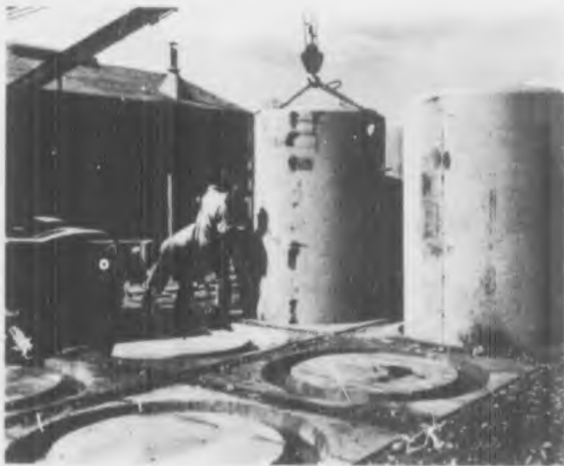
Figure 2. Placing a concrete cylinder during test section construction
