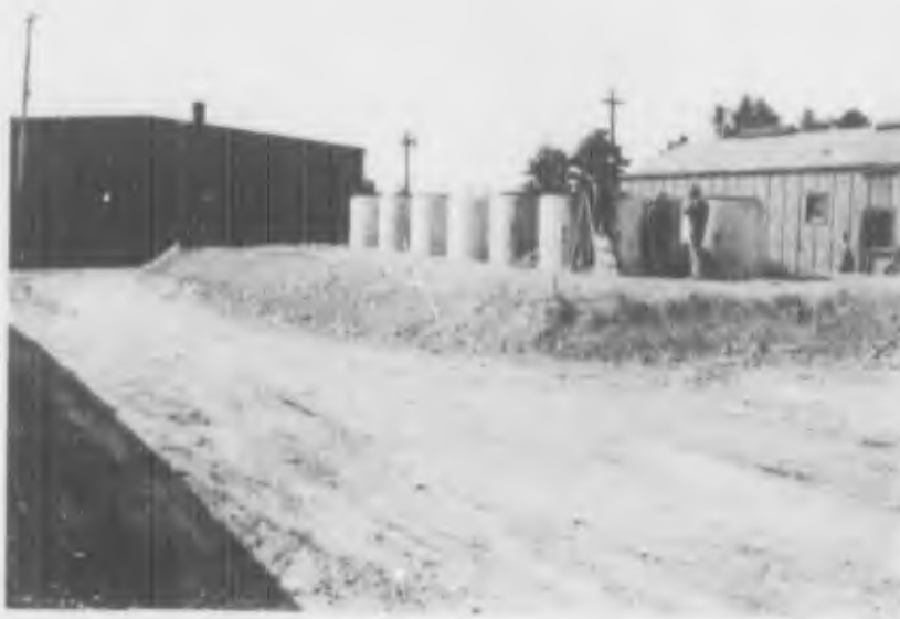
Figure 1. All concrete cylinders and gravel backfill in place
