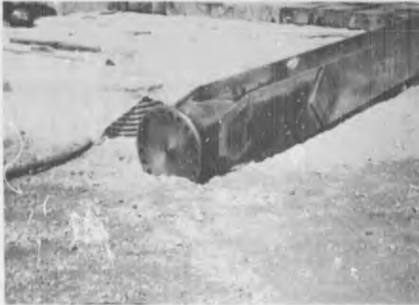
Photo 4a - Head Attachment for Driving H-Piles with the Bodine Sonic Hammer
