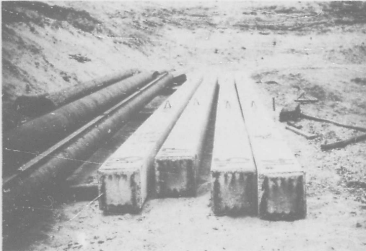
Photo 1a - Timber, Steel Pipe, and Prestressed Concrete Piling at Site
