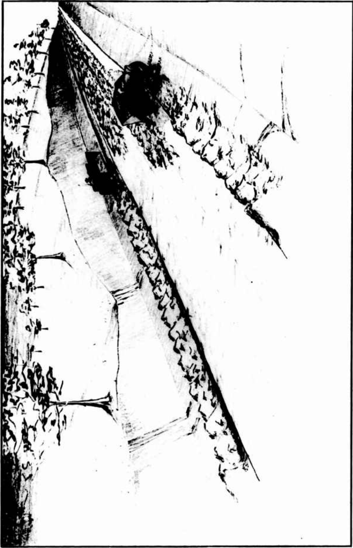
Fig. 6. Replacing soil on lower membrane
