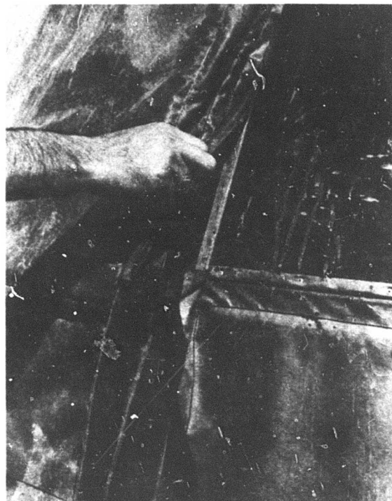
Figure 88. Final Attachment of Arch Beam Flashing
