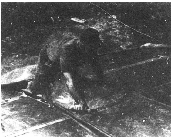
Figure 87. Straddle Position for Attachment of "Quick-Edge"
