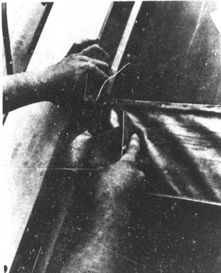
Figure 35. Use of Flashing Tool
