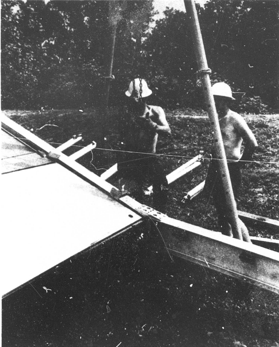
Figure 37. Lifting the Arch
