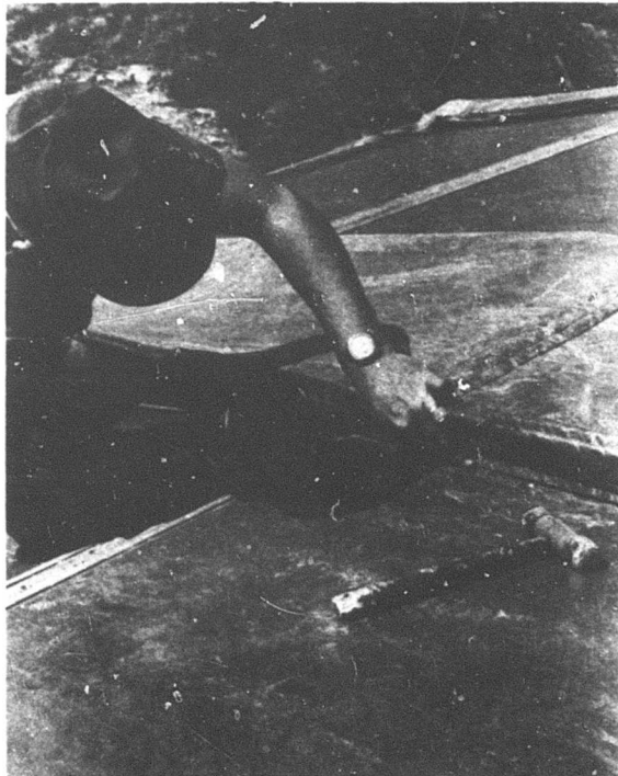
Figure 86. Attachment of "Quick-Edge"
