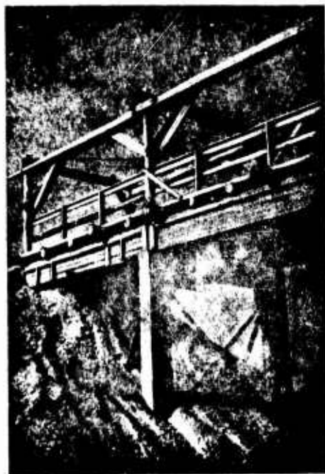
Fig. 227. A view of a sectional ferroconcrete trestle.
