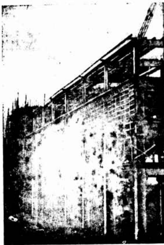
Fig. 283. View of a ferro-concrete loading hopper with a suspended parabolic capacitive part.
