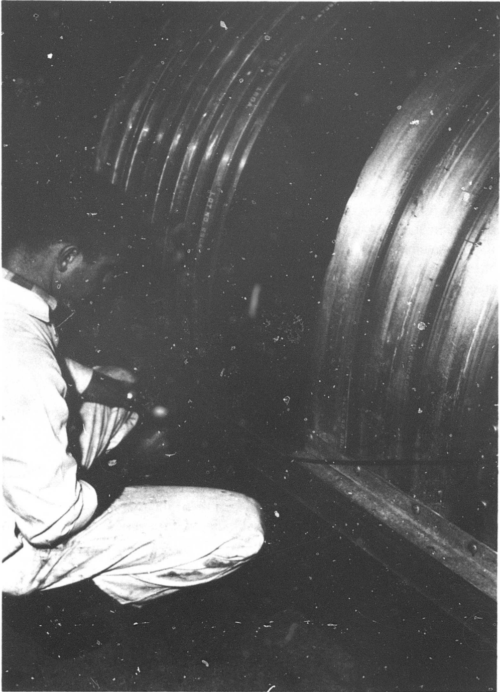
Figure 9. Heat-shrinkable polyethylene band being applied over arch joint.
