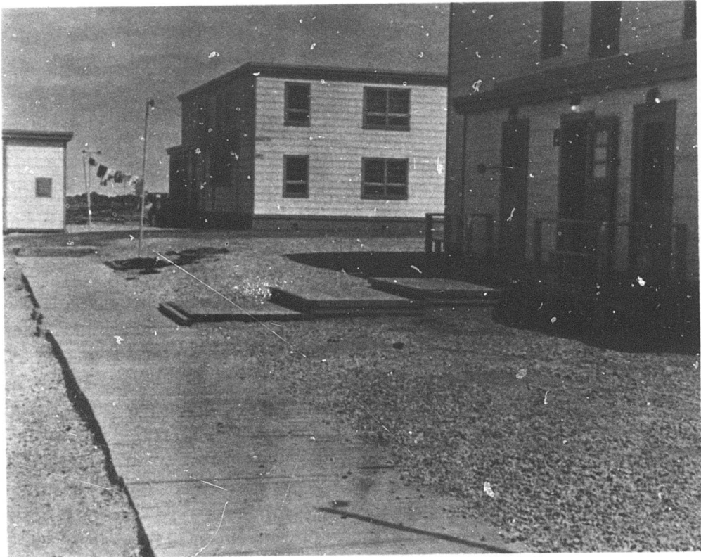
Figure A-6. Utilidor under entry to building at Fort Churchill.
