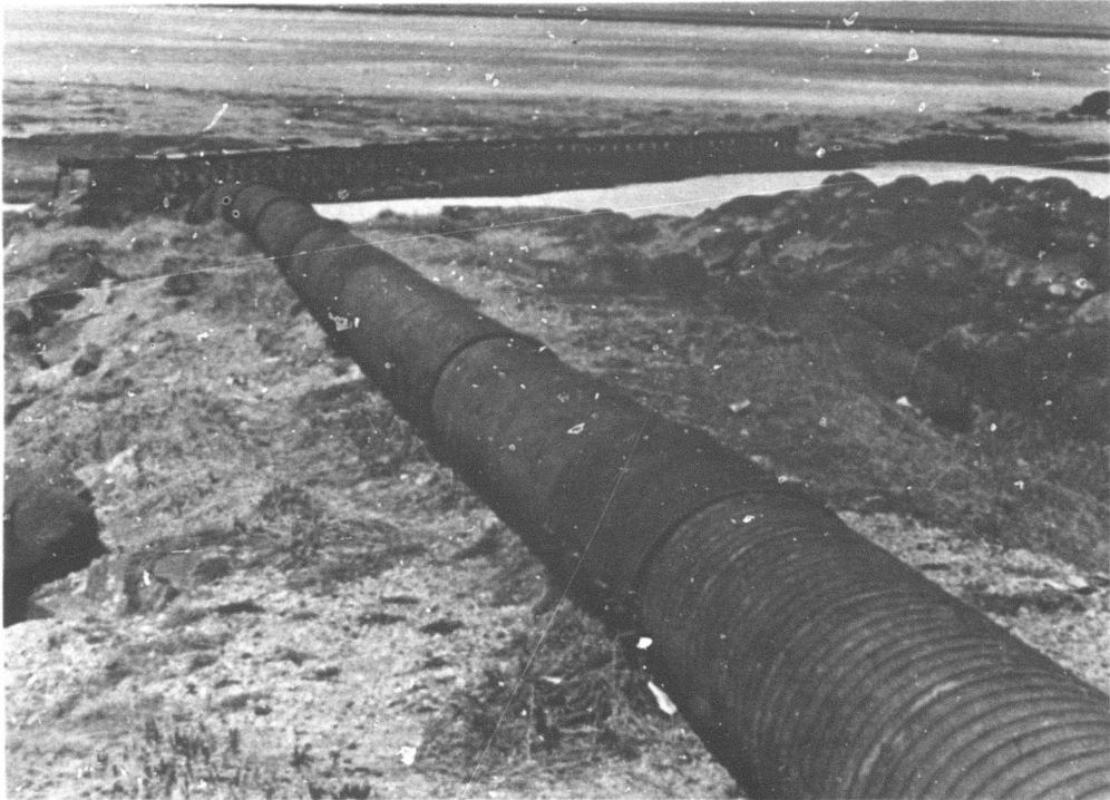
Figure A-8. Sewage outfall line and outfall house at Fort Churchill.
