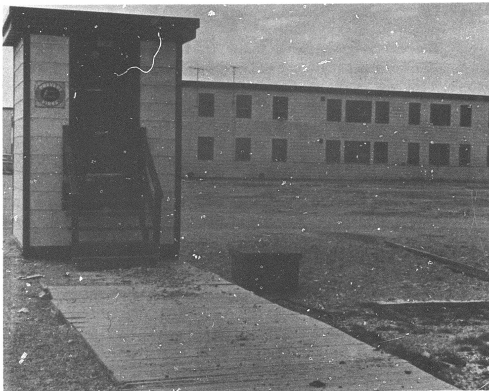
Figure A-7. Fire hydrant in small house over utilidor at Fort Churchill.
