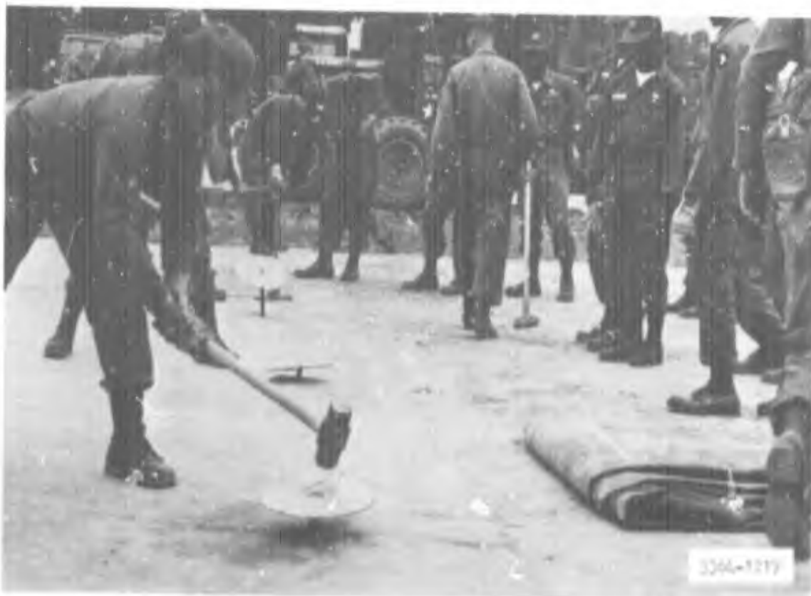
Photograph 1. Guy anchors driven into soil subgrade with sledgehammers
