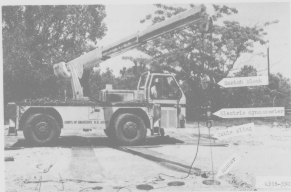
Fig. 9. Mobile crane used to remove anchors from the soil subgrade
