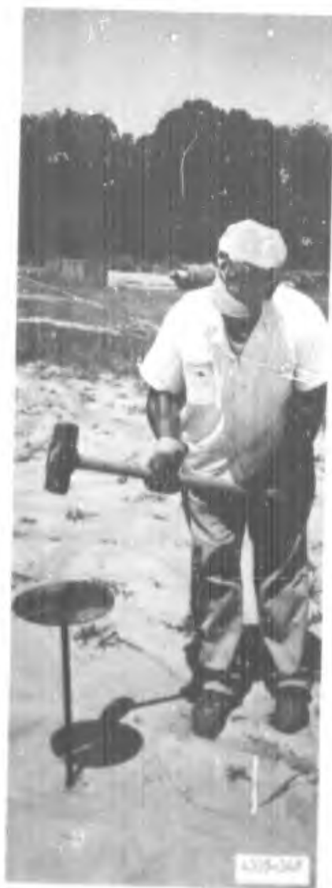
Photograph 22. Driving guy anchor into subgrade with sledgehammer
