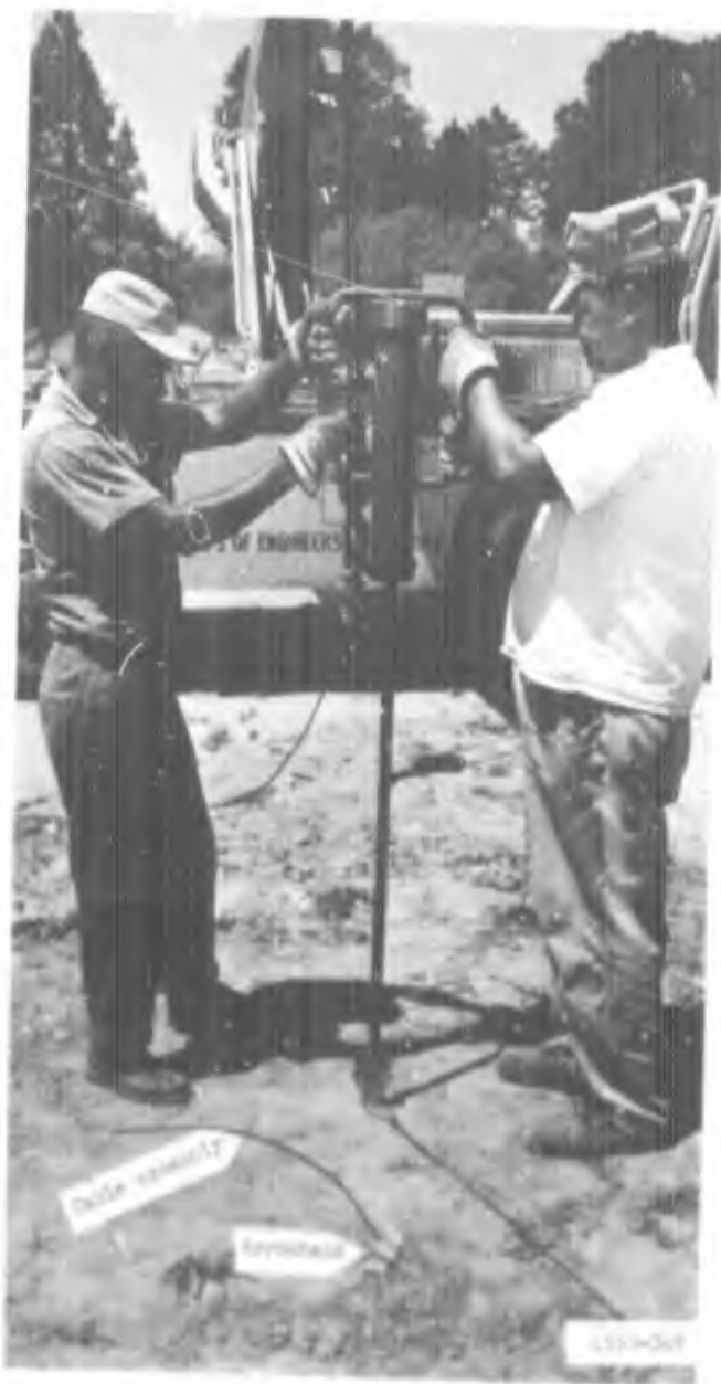
Photograph 21. Driving arrowhead anchor into subgrade with manual impact tool
