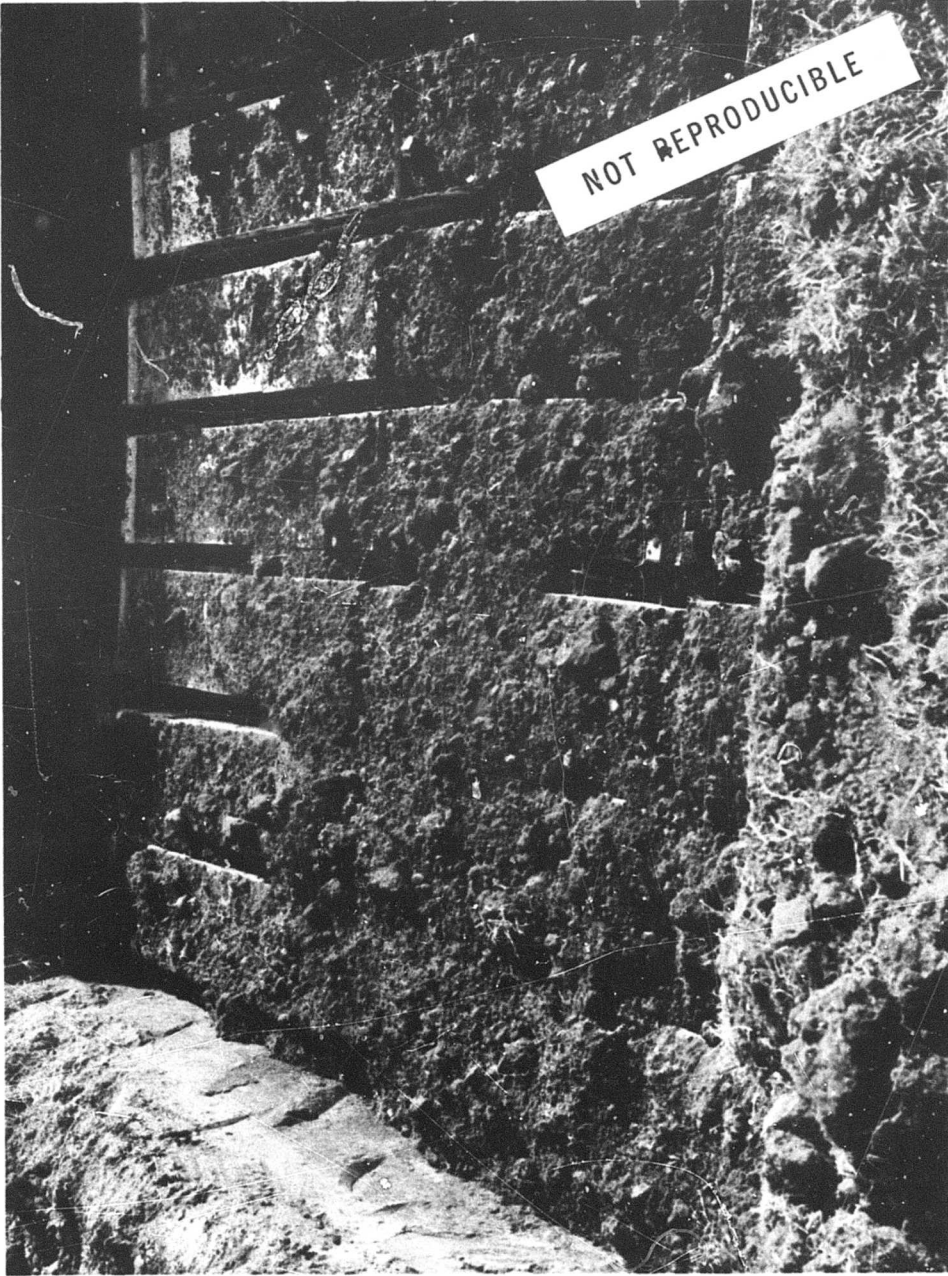
Figure C-1. Beams being buried for deterioration tests.
