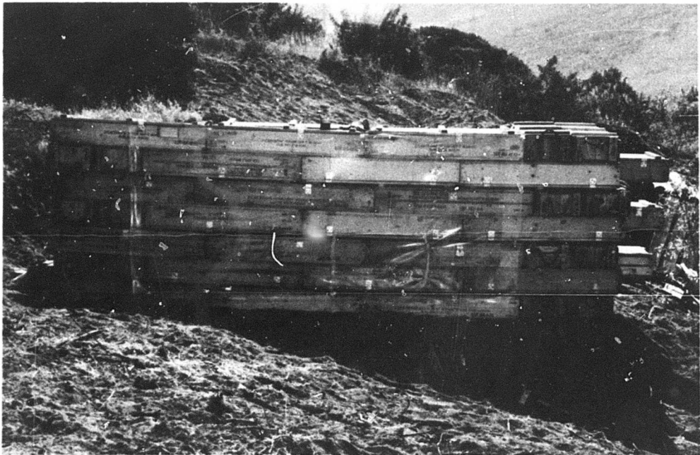
Figure F-2. Test wall simulating bunker.
