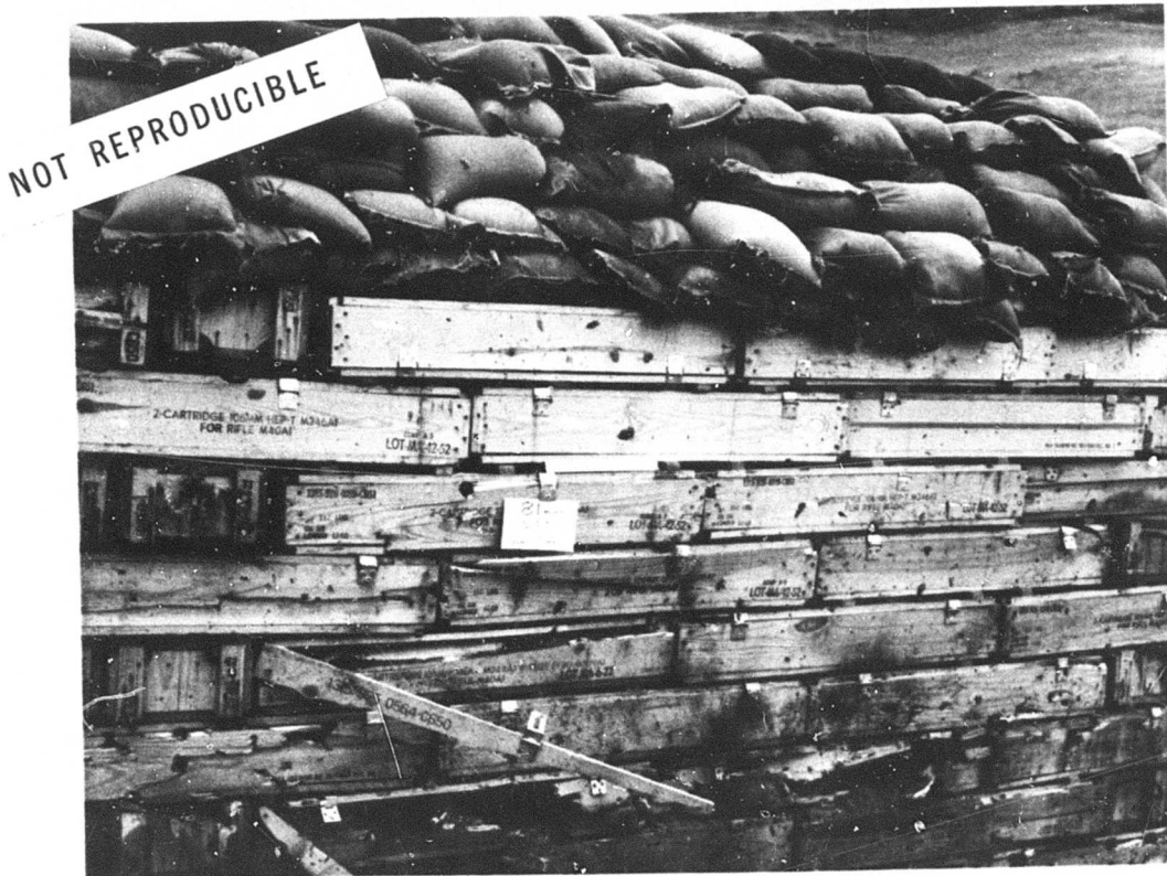
Figure F-7. Damage from 81-mm round at 4 feet.
