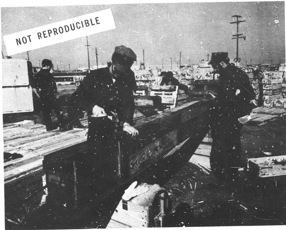
Figure E-5. Overhead beam construction.
