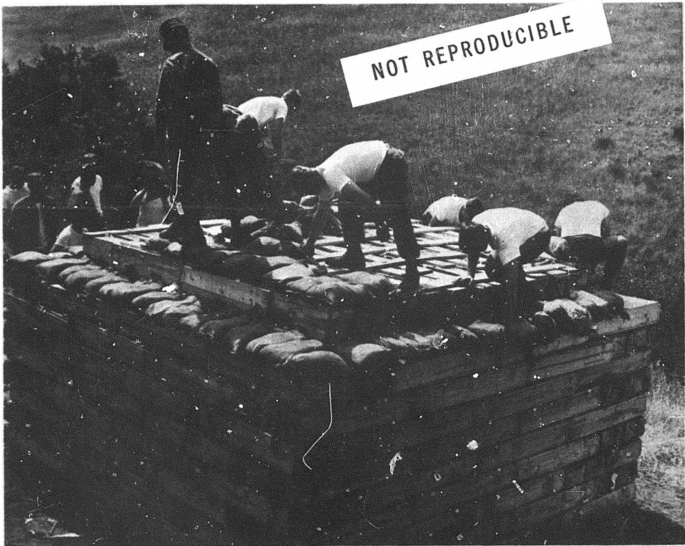
Figure F-1. Bunker construction at Camp Pendleton.
