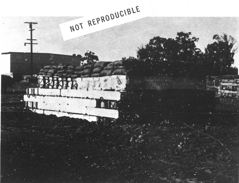
Figure E-10. Oblique view of bunker.
