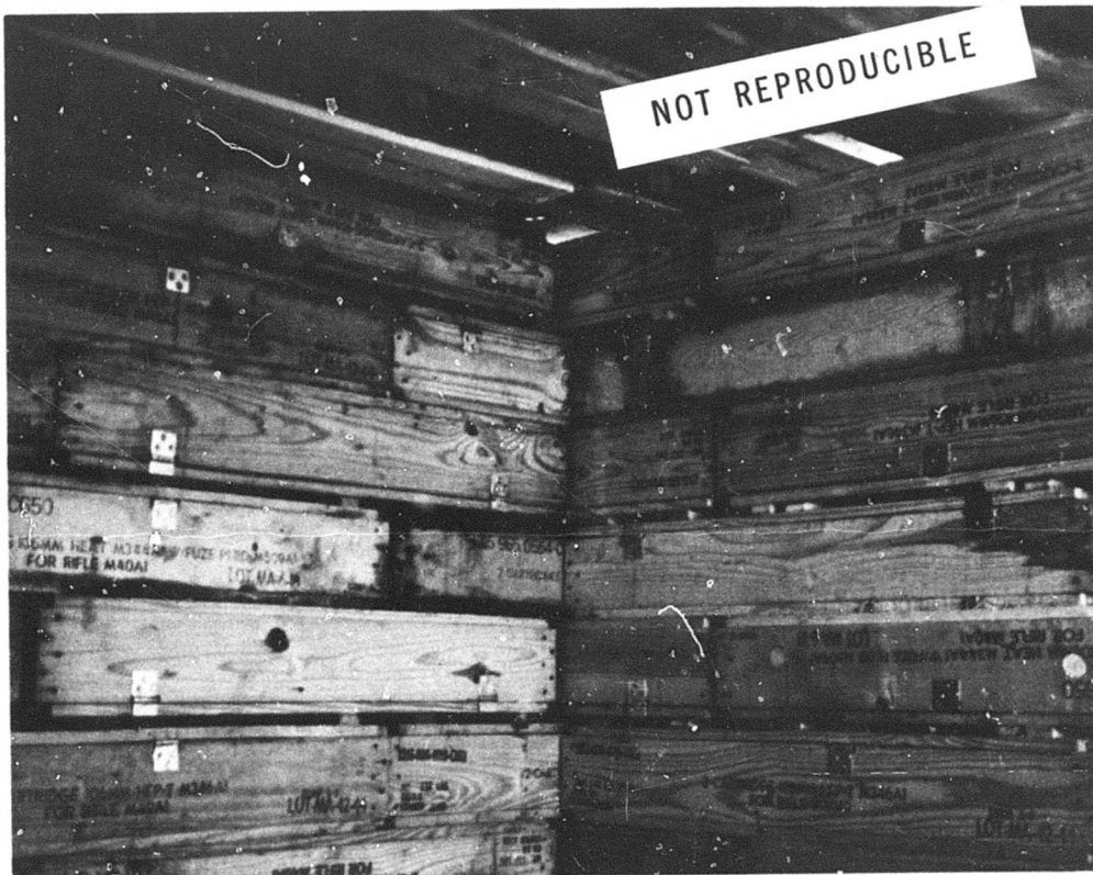
Figure E-8. Interior of bunker.
