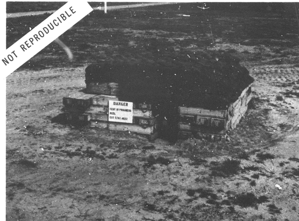
Figure 9. Bunker constructed with 106-mm ammunition boxes.
