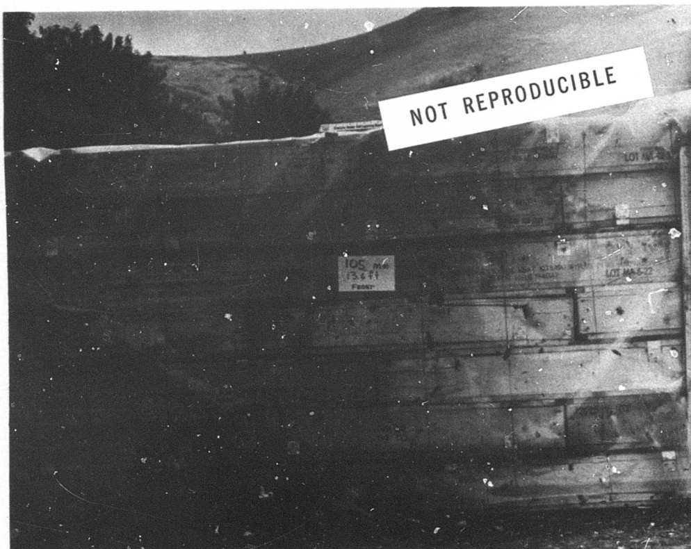
Figure F-8. Damage from 105-mm round at 13.6 feet.
