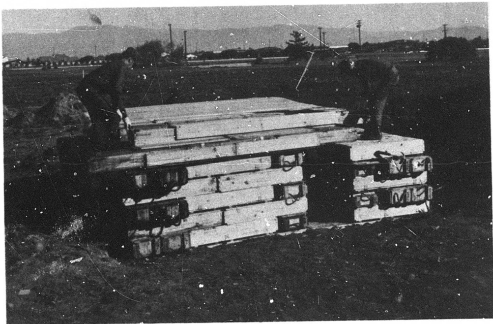
Figure E-6. Placing overhead beams in position.
