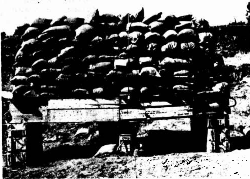
Figure 5. Field load test of beams.
