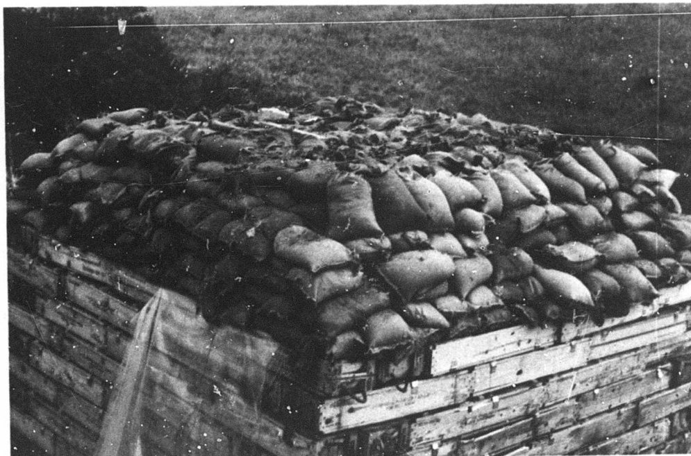
Figure F-9. Damage from 81-mm round 2 feet above roof.
