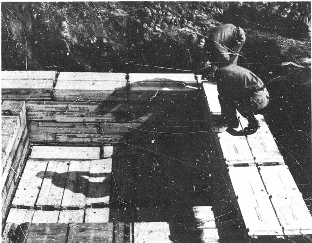
Figure E-4. Bunker wall construction.
