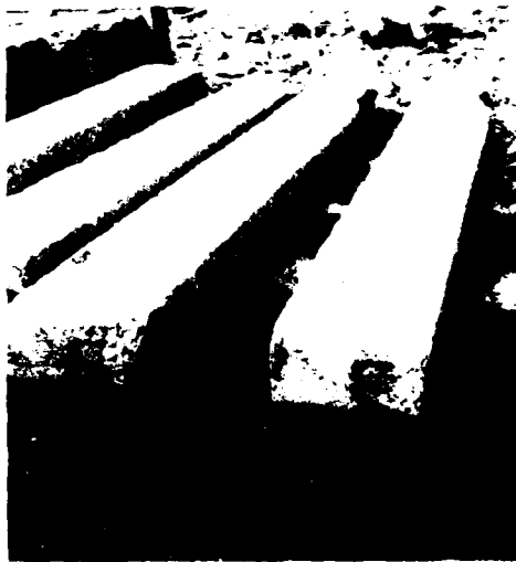
d. Beam 8, seaward end
