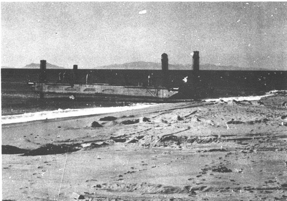
Figure 8. Ammi pontoon lifted out of surf by block and tackle gear.
