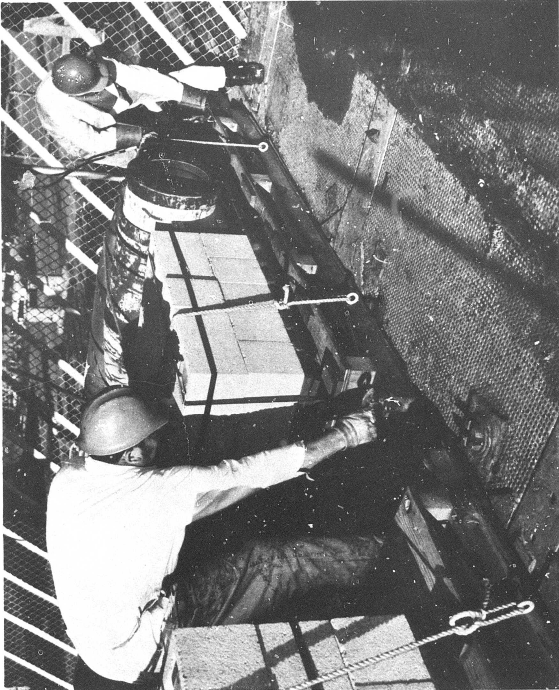
Figure 6. Hooking up a NCEL large pallet for crane off-loading.
