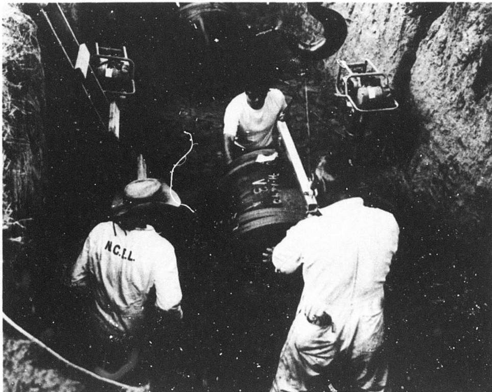
Figure 16. Lowering of model CN-1 on soil bed with crane.
