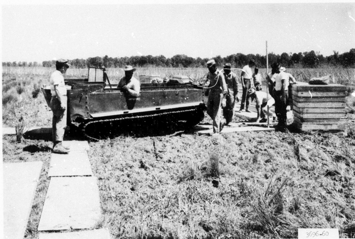
Photograph 20. Tracked vehicle (Weasel) used to tow mat bundles to assembly area. Mat from previous investigations (foreground) used for walkway
