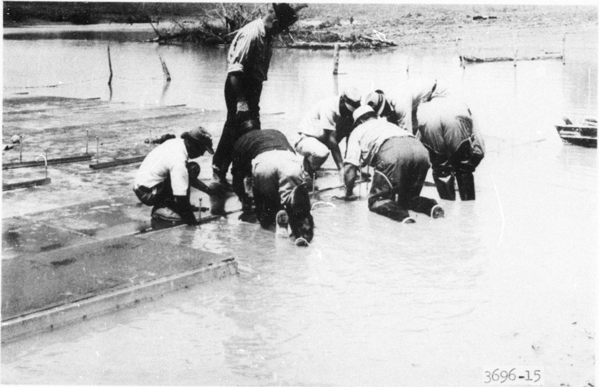
Photograph 9. New panel being forced underwater in order to connect it to pad
