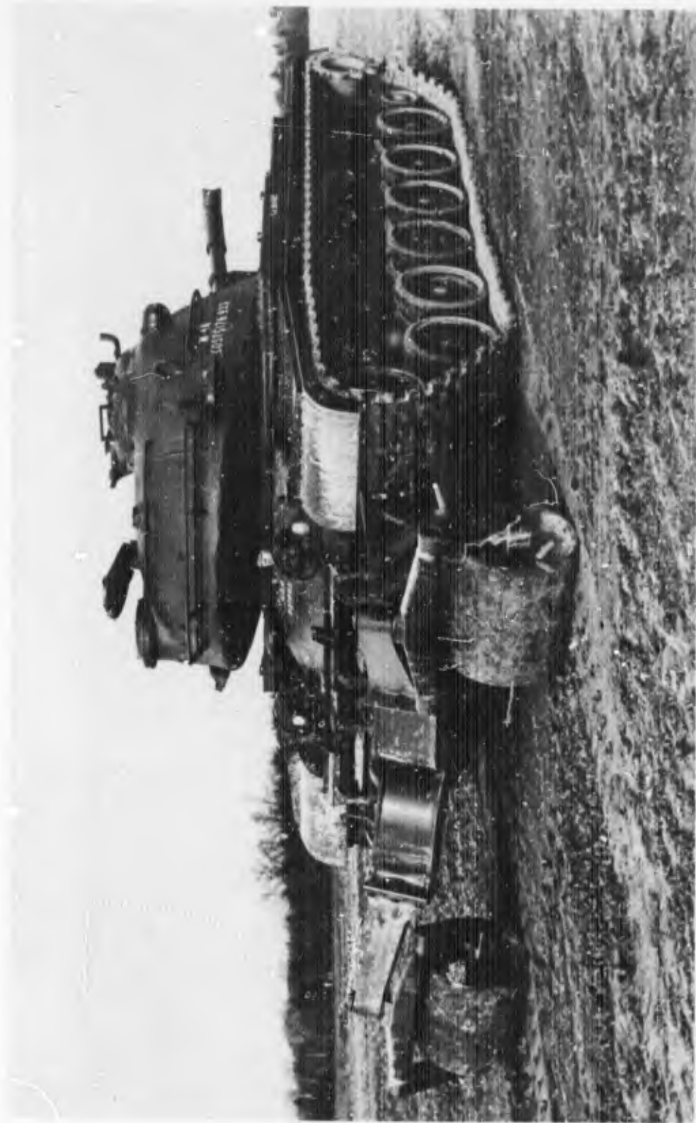
Fig. 1. The original expendable, mine-clearing roller (Model I).
