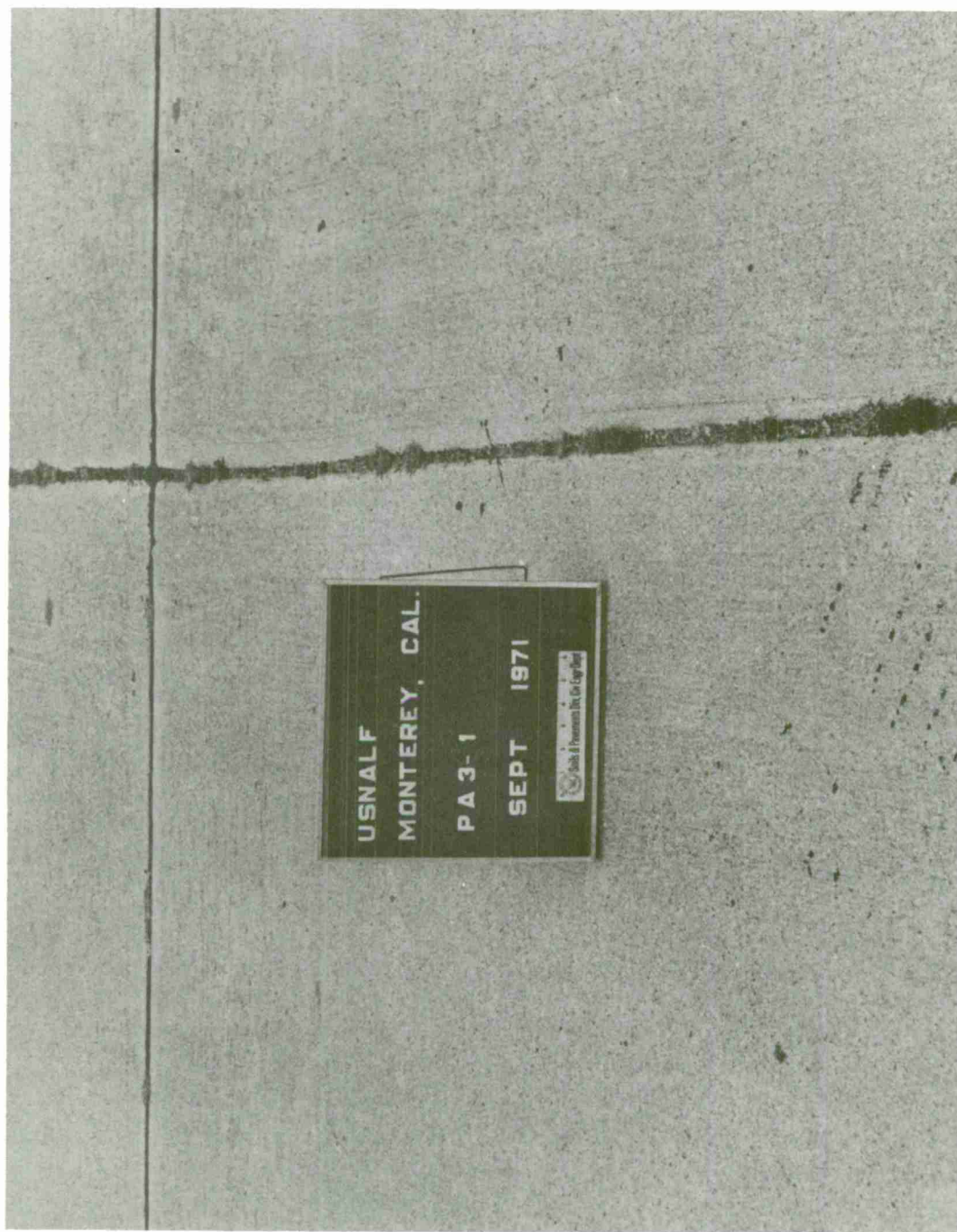
Figure 19. Vegetation growing through joint, Discrete Area PA3-1.
