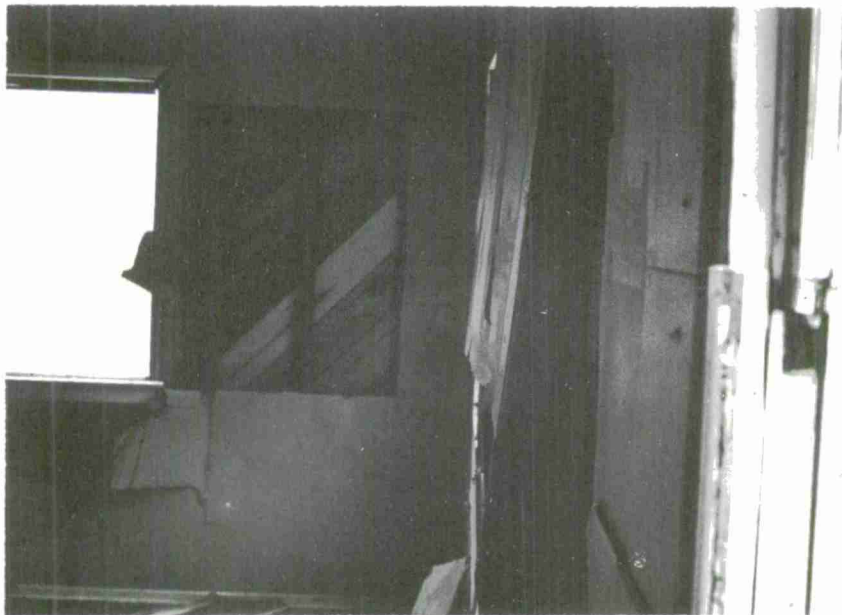
Fig. B-2. Posttest Living Room, North Wall Looking West
