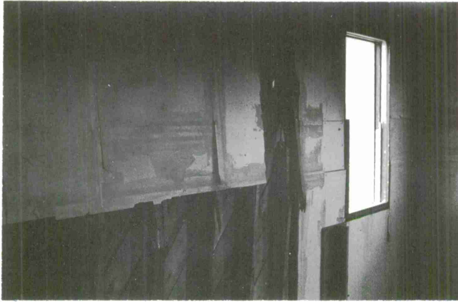
Fig. B-1. Posttest Living Room, North Wall Looking East
