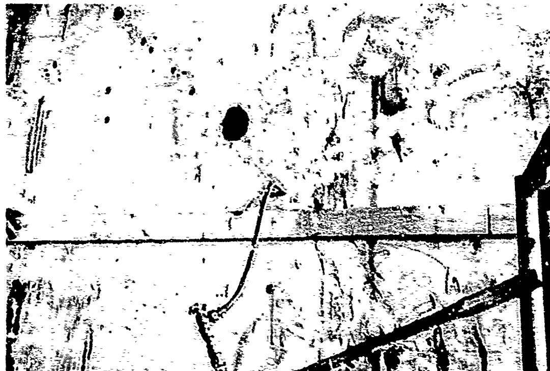
Fig. 3. Close-up of R wall, main lobby, showing sealer, grouting nozzle, and core holes
