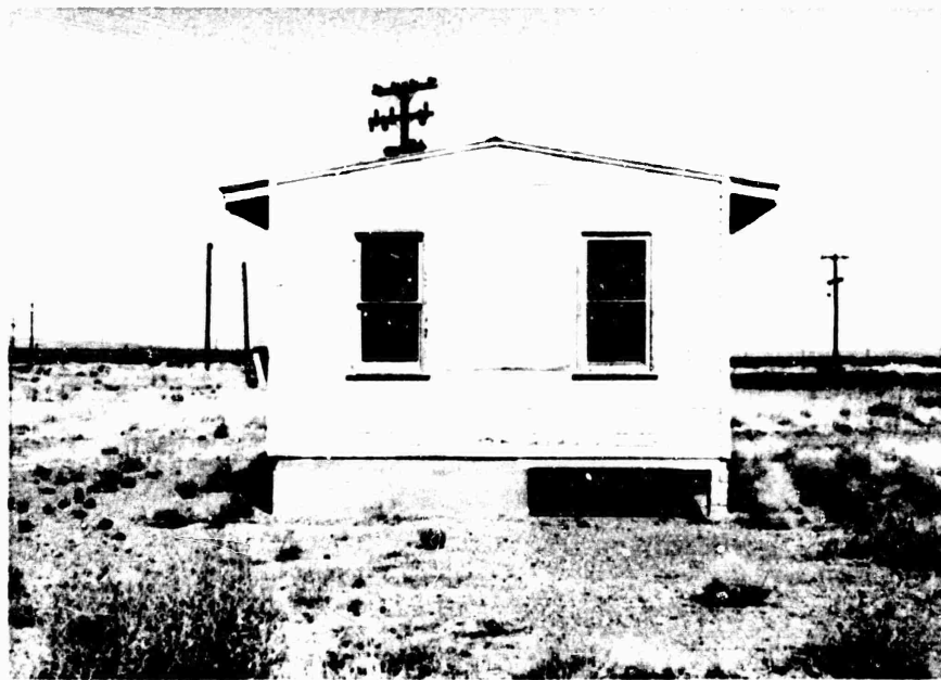
Fig. 30 W-4, Southerly Exterior
