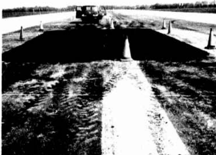
Photograph 6. Area on runway 18-36 that was patched after failure from C-130 operations
