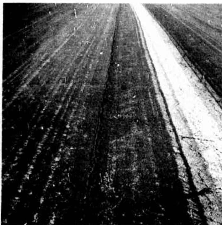
Photograph 4. General condition of surface of pavement that was not overlaid in 1967
