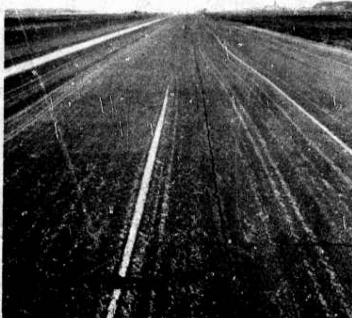
Photograph 3. Longitudinal joint opening and shrinkage cracking in parallel taxiway
