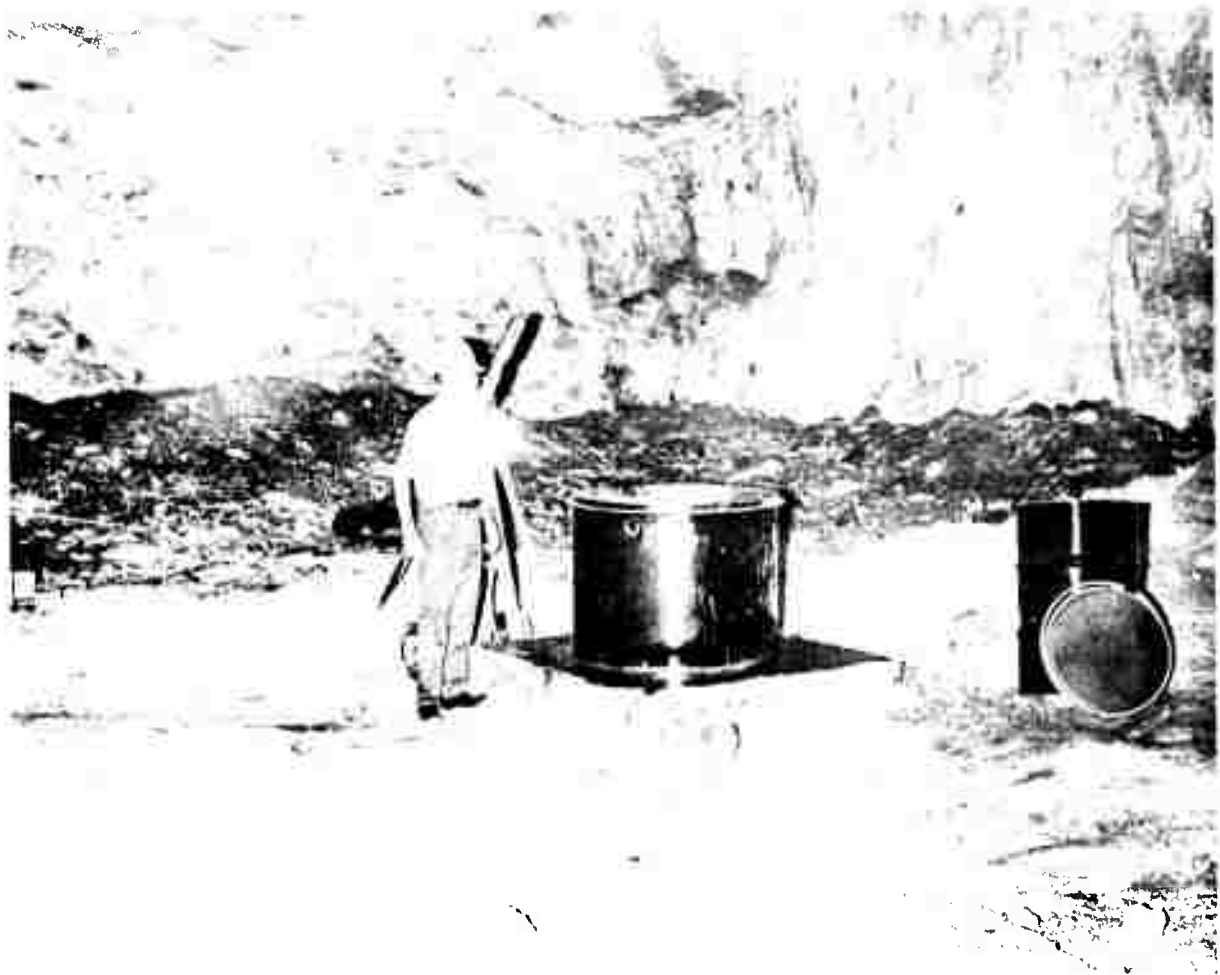
Figure 98. Completed vault installation in Kleer Mine, Grand Saline, Texas (GA3TX)
