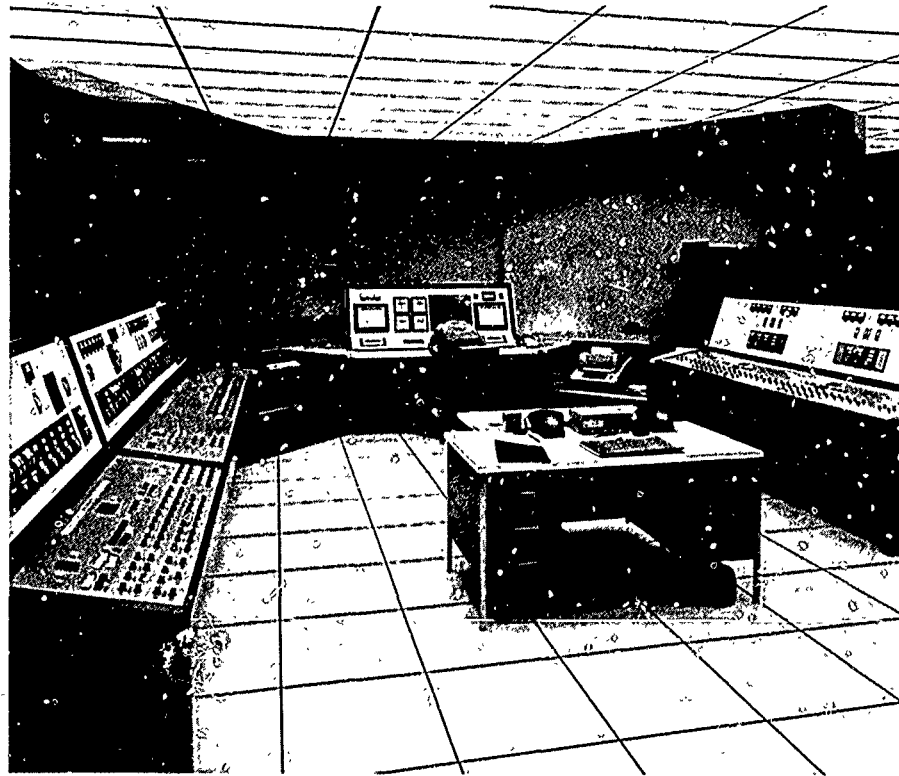
FIGURE 4.105 Lone Star Cement Control Center, Greencastle. [Photograph courtesy of Leeds & Northrup Company.]
