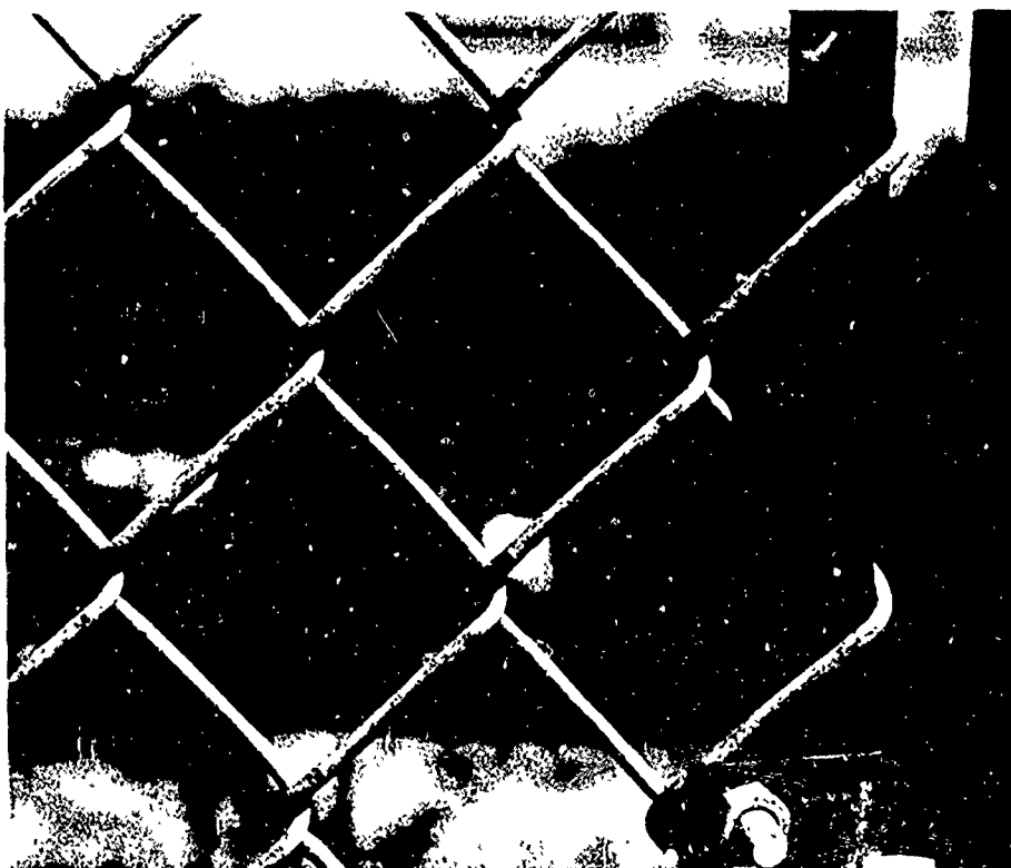
Figure 3. System 1. Newly installed zinc coated steel.
