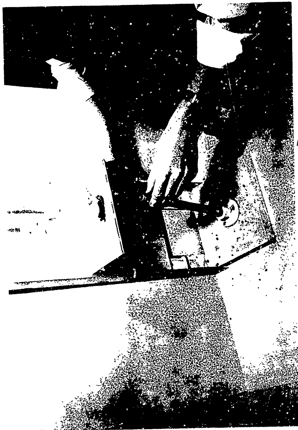
Fig. 6. Removing tiled coaxial line
