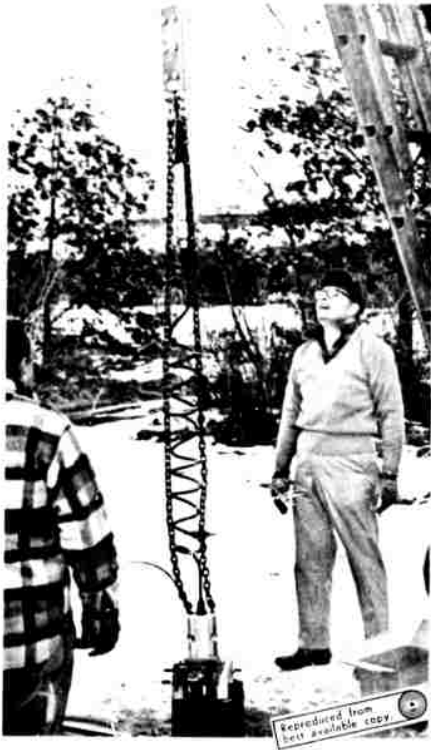
FIGURE 1. VIEW OF CHAIN-TYPE CABLE DECOMPRESSION
