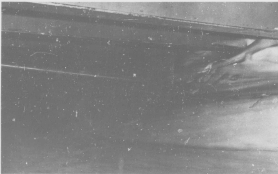
Figure 3. Utility pipes beneath Building 155 becoming engulfed in drifted snow.
