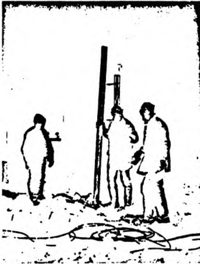
Fig. 2. The "Annemirl" Is Ready for Operation. The bottom part (with copper jacket) contains a heating element and measuring instruments; the long epoxy tube contains the winding reel and the oil tank.
