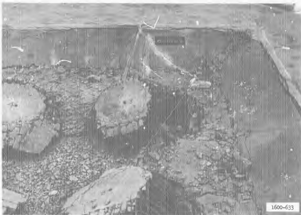
b. Northwest corner of the slab.
