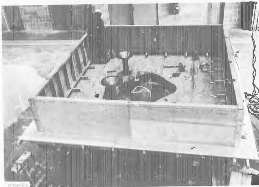
b. Overhead view of inner wall forms.
