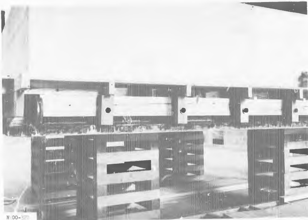
a. Base of wall forms.
