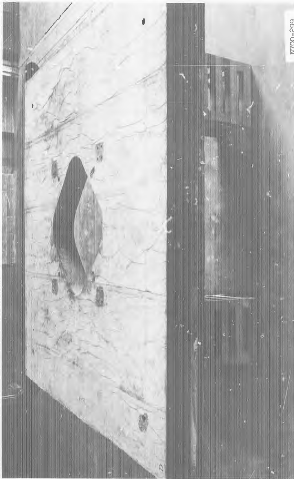
Figure 3.4 Base slab ready for start of model formwork construction.
