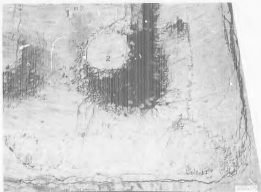
b. Northeast slab corner.
