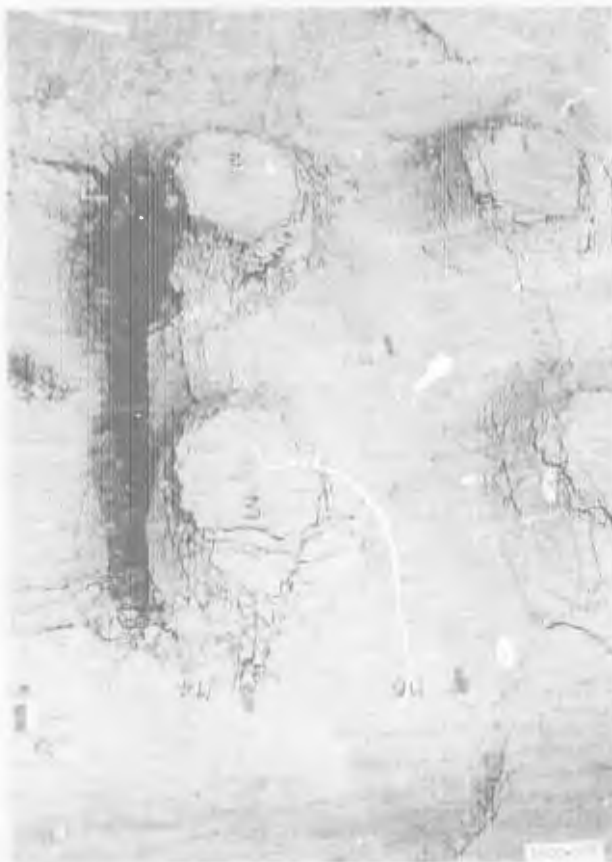
a. Center of slab from west side
