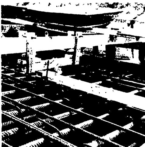
b. Timber support with soil stress meter S-14 attached in position prior to placement of concrete
