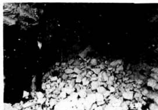
c. Muck pile after about 20 shots
