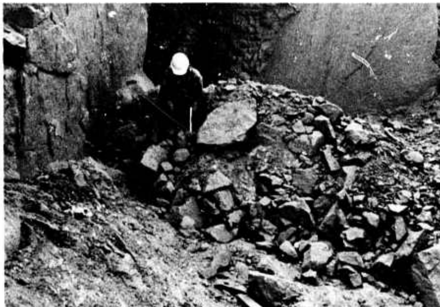
a. Typical muck pile after removal from tunnel; note occasional large boulder
