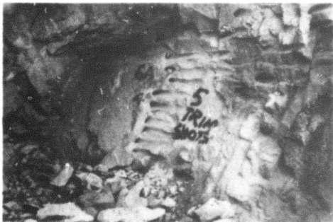
b. Flat surface is formed using 5 shots with the 57 mm gun
