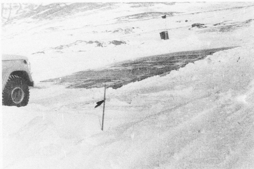
Figure 3. Timber ramp constructed during DF-68 at sea ice to land transition.
