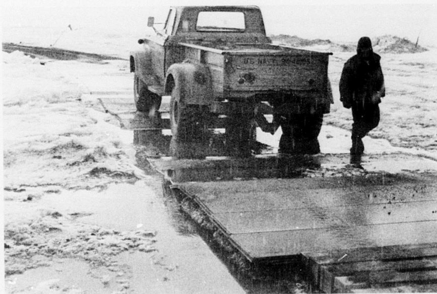
Figure 12. AM_2 aluminum planking after melting occurred.
