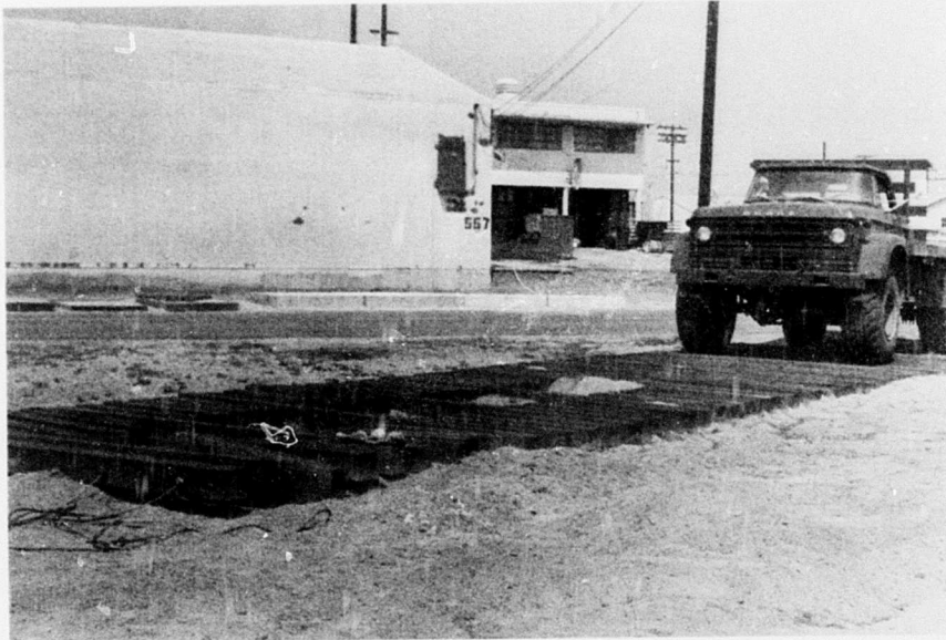
Figure 7. Dodge W-500 traversing prototype timber ramp on beach sand.
