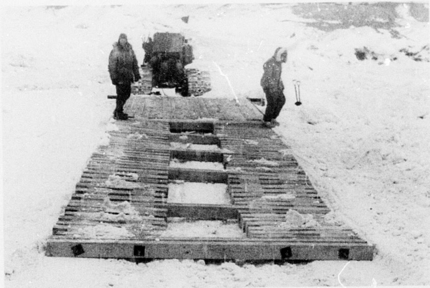
Figure 9. Timber test sections being moved into place.
