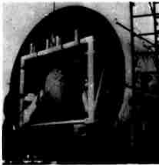
Figure 7. Hydrazine gas-generation system being installed in pontoon.
