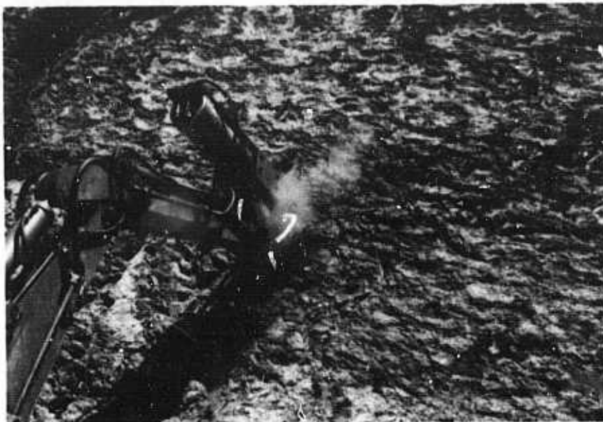
Plate 7 Progress of Excavation
