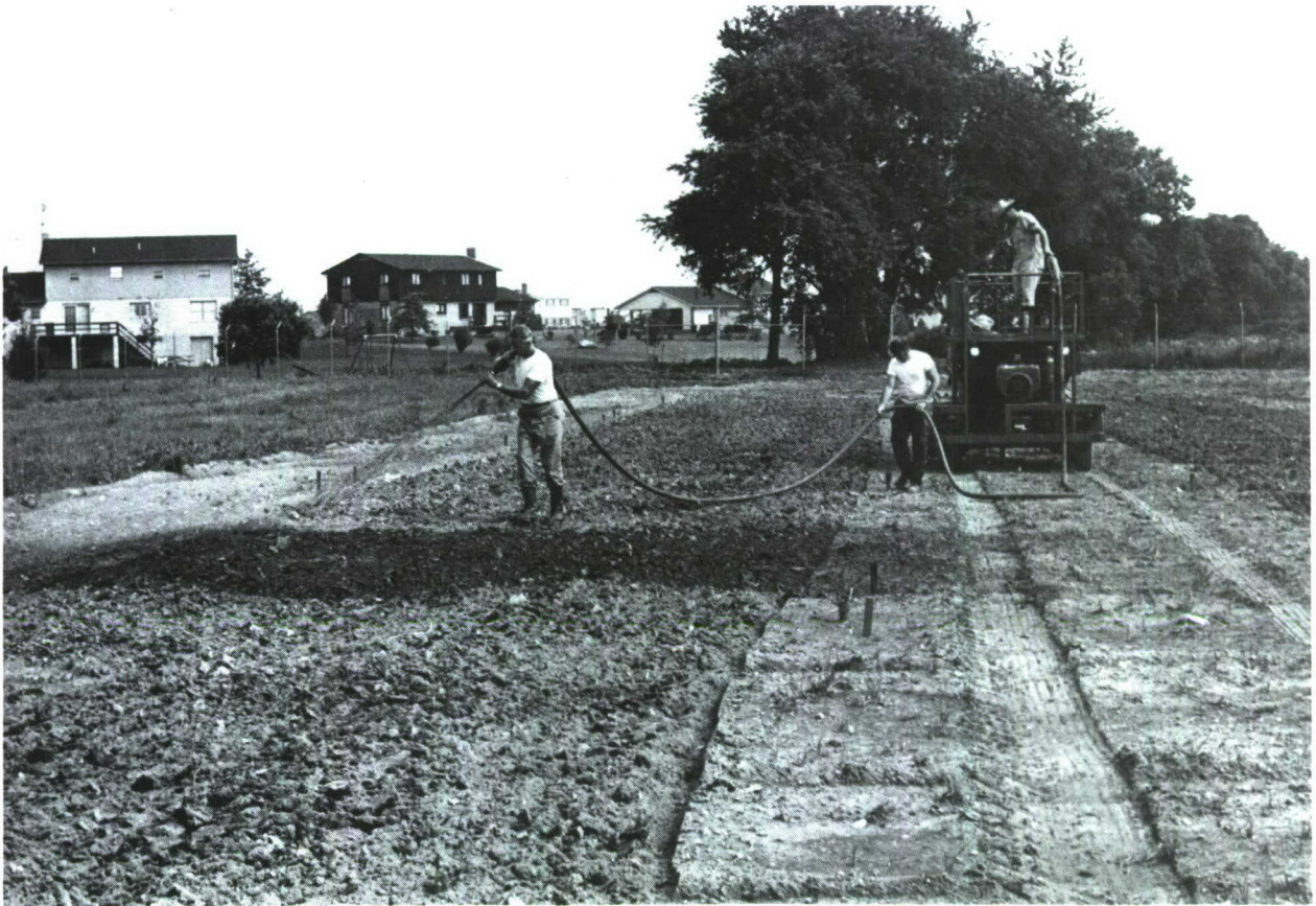
FIGURE 20. Field Test 3 - Bowie Hydromulcher during spray application with hose.
