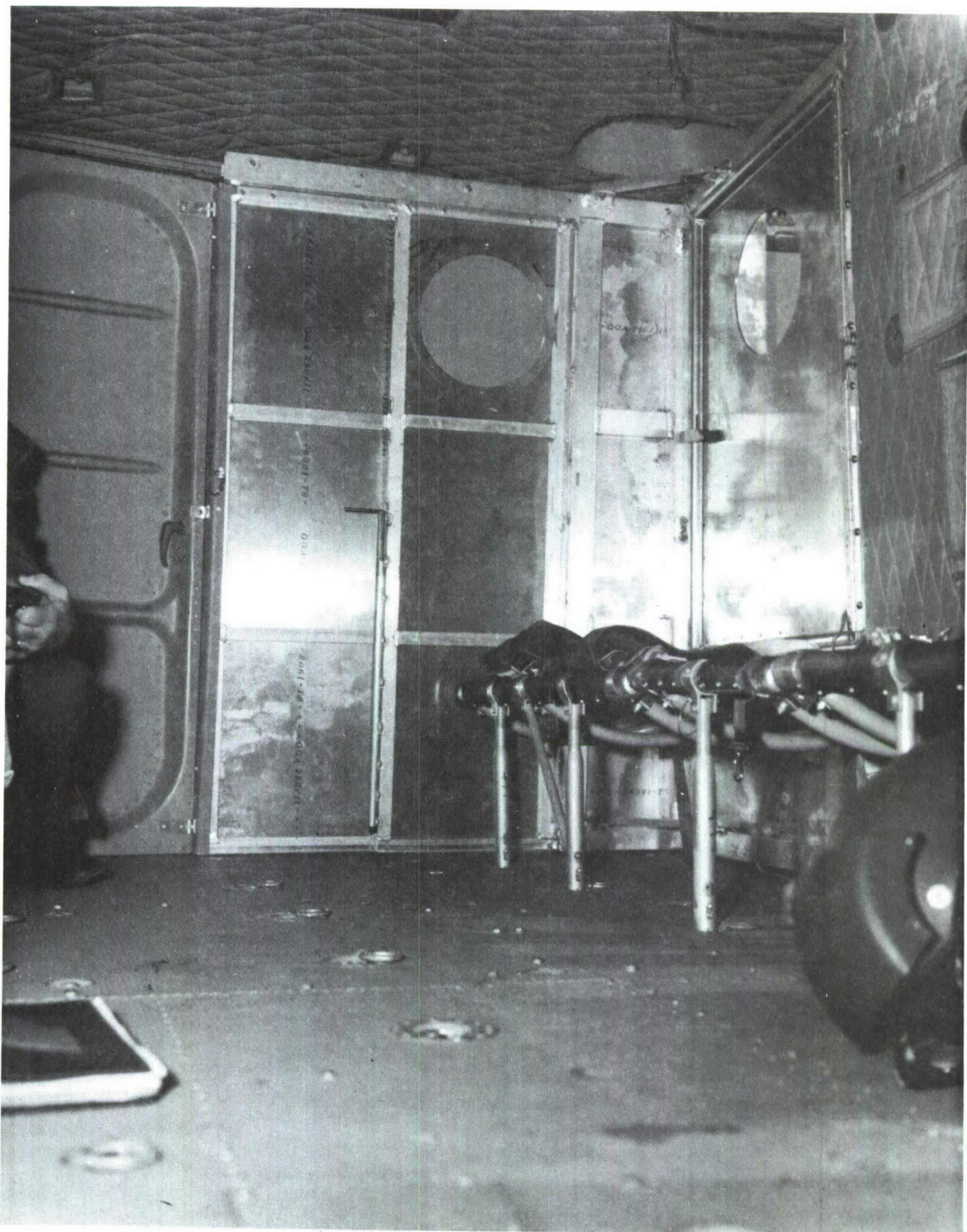
Figure 5. Interior View Showing L Hanger For Sliding Doors
