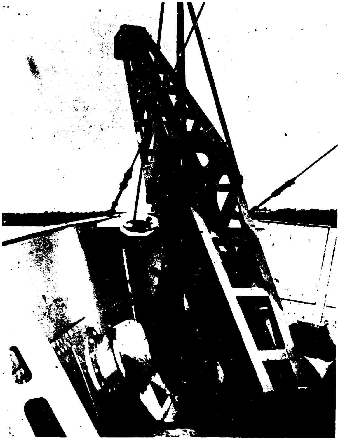
FIGURE 1 MOUNTING STRUCTURE FOR TRANSDUCER PACKAGE
