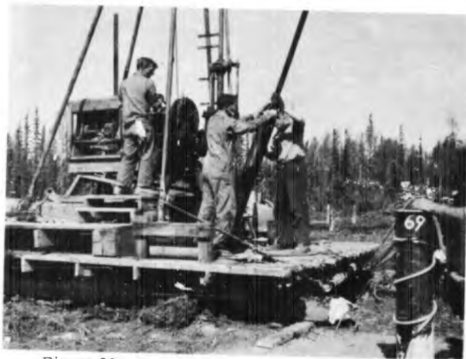
Figure 20. Core barrel used with Longyear drill.
