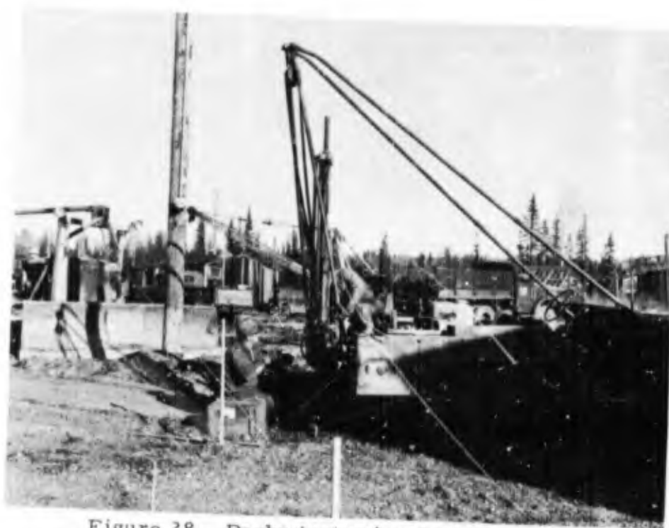
Figure 28. Probe test using Acker core drill.
