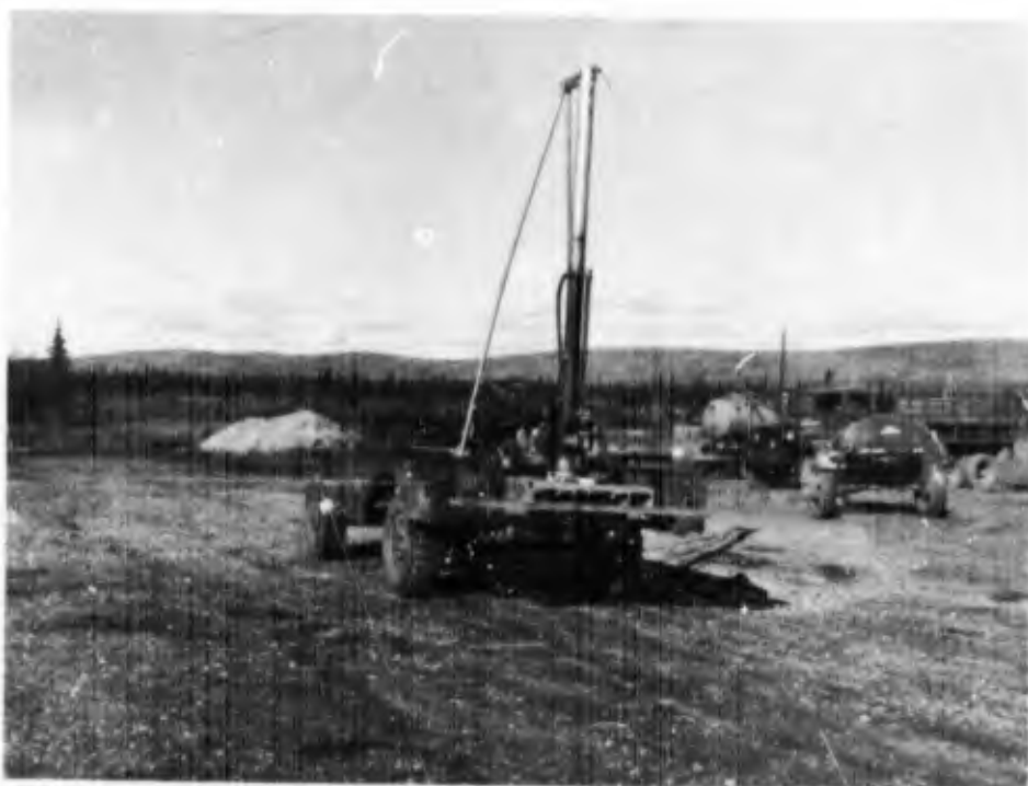
Figure 32. Concore core drill mounted on 3/4-ton truck.
