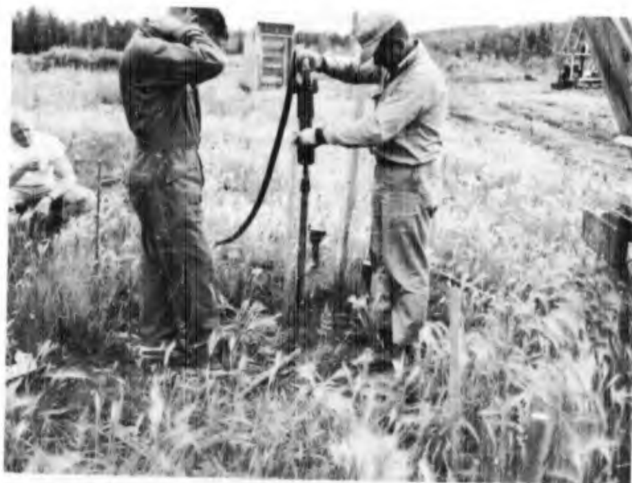
Figure 56. Driving Shelby tube with pavement breaker.
