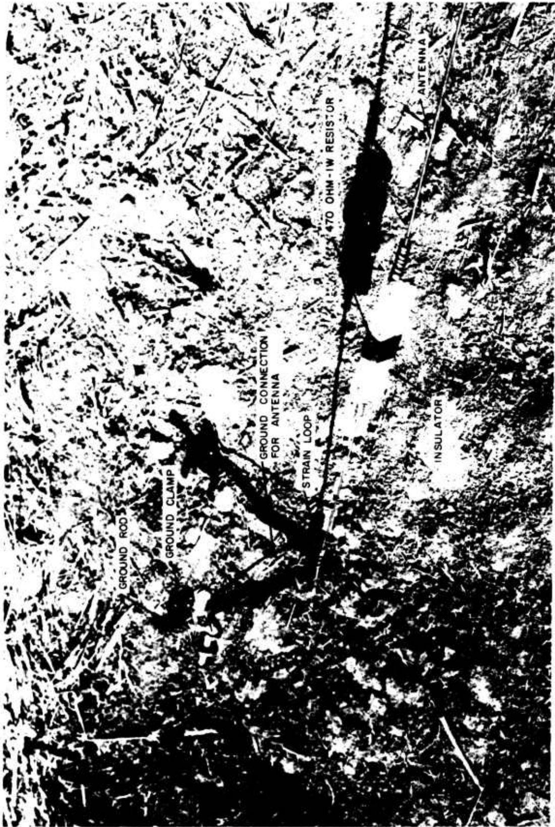
FIGURE 10. DETAILS OF TERMINATION AT OUTER RADIUS
