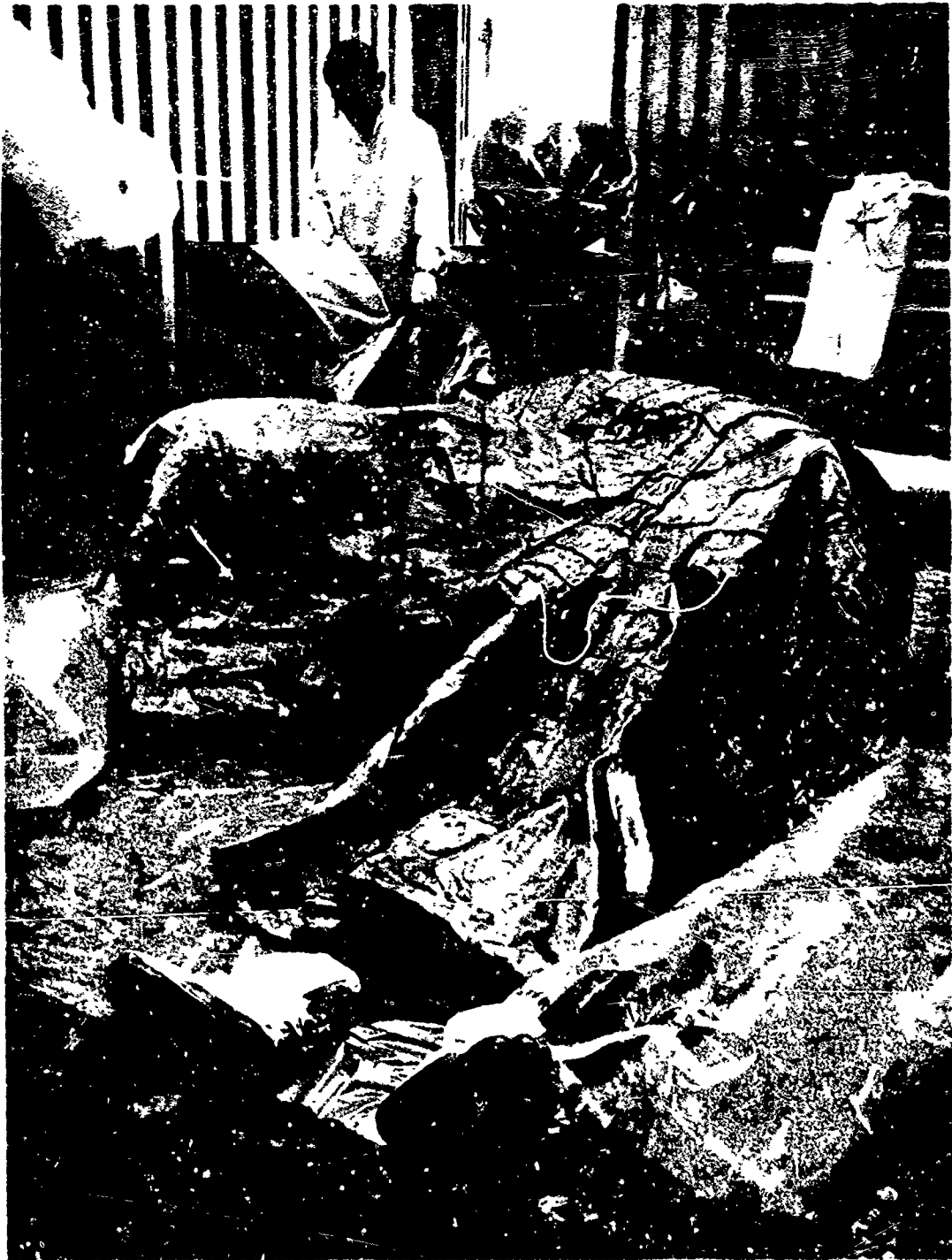
Figure 180. Removing Form Tool Segments from Within Welded Apex Cross Ply
