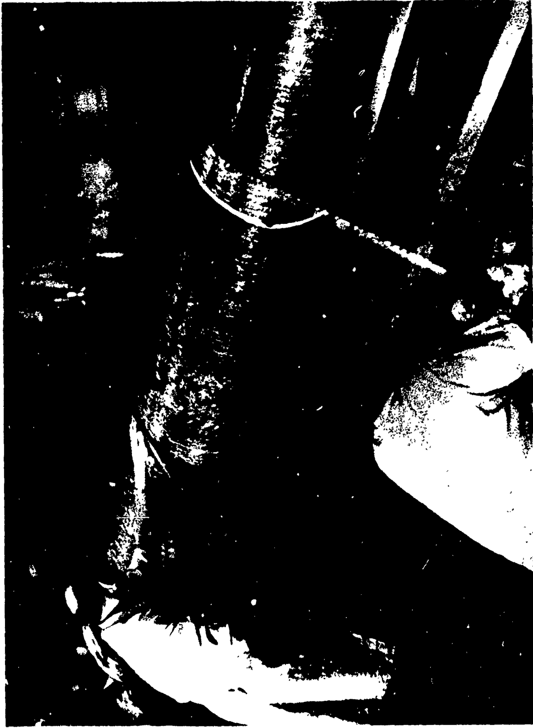
Figure 150. Wrapping Impregnated Boom with Shrink - Tape
