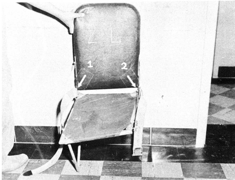
Fig. 45. Both aisle floor attachments of seat 2L tore completely free. The seat was forced in a forward direction, partially "hinging" at its two wall attachments, which were badly distorted. The safety belt showed evidence of incipient failure near its attachment, and both the left and the right brackets joining the seat pan and the seat back were badly distorted (arrows 1 and 2).
