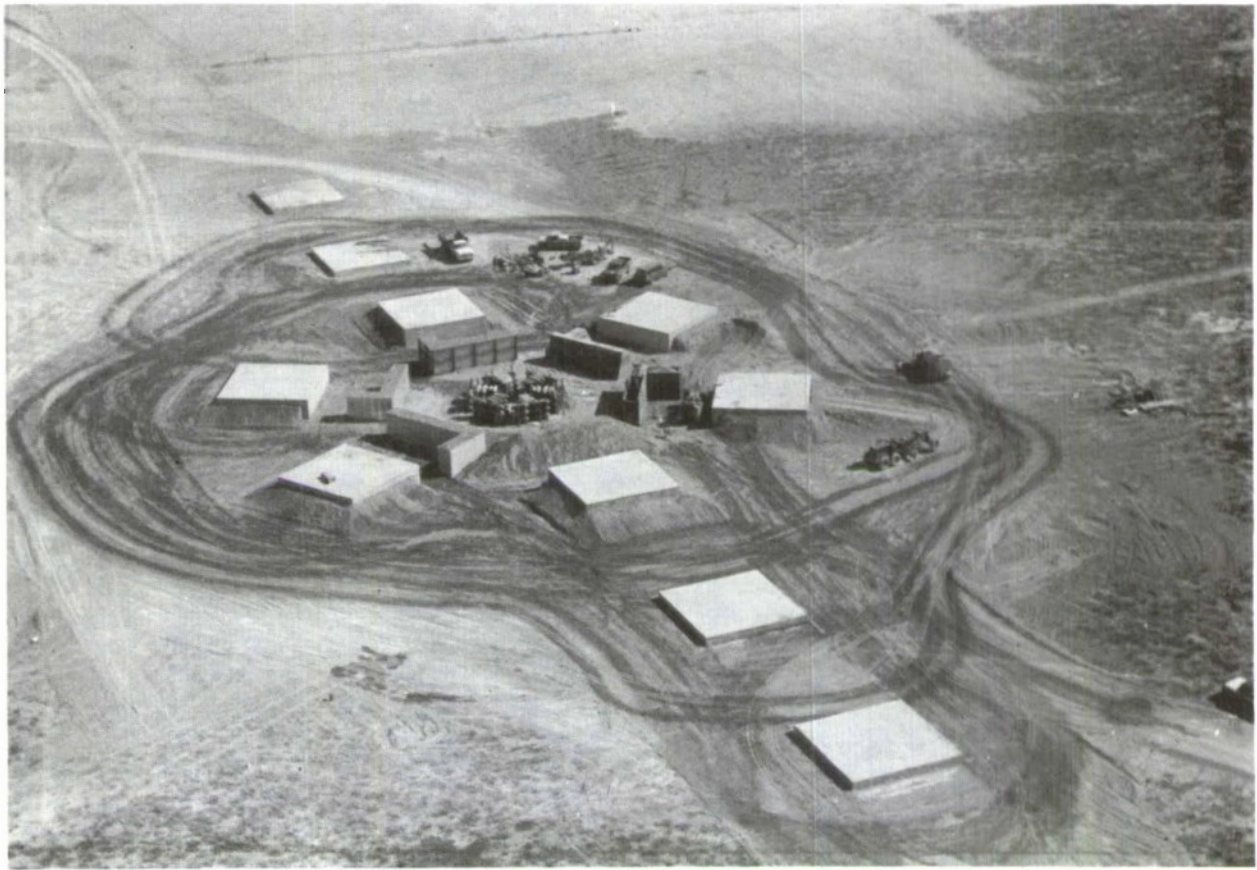
Figure 36. Aerial View of Phase III Test Configuration
